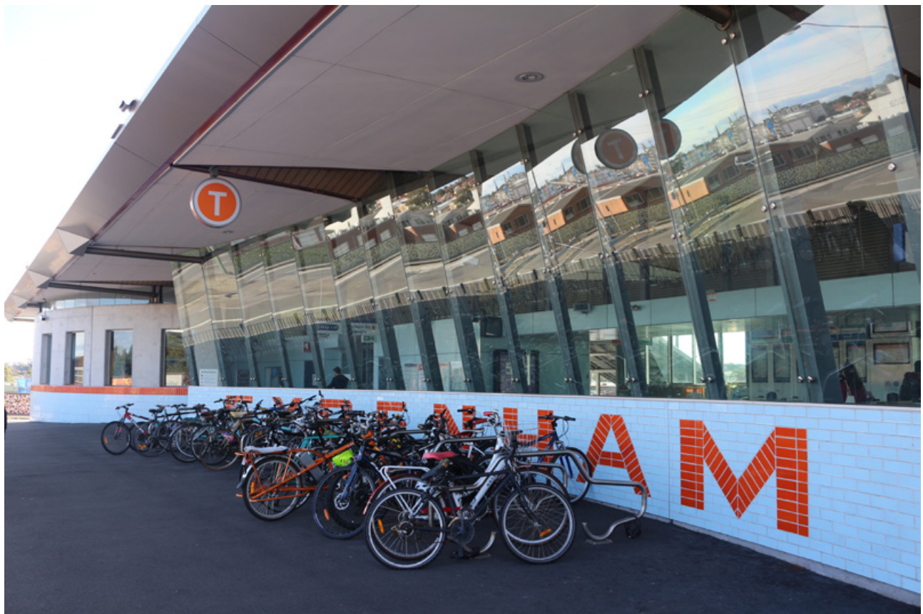
Plate 16-2 Sydenham Station entrance at Gleeson Avenue
