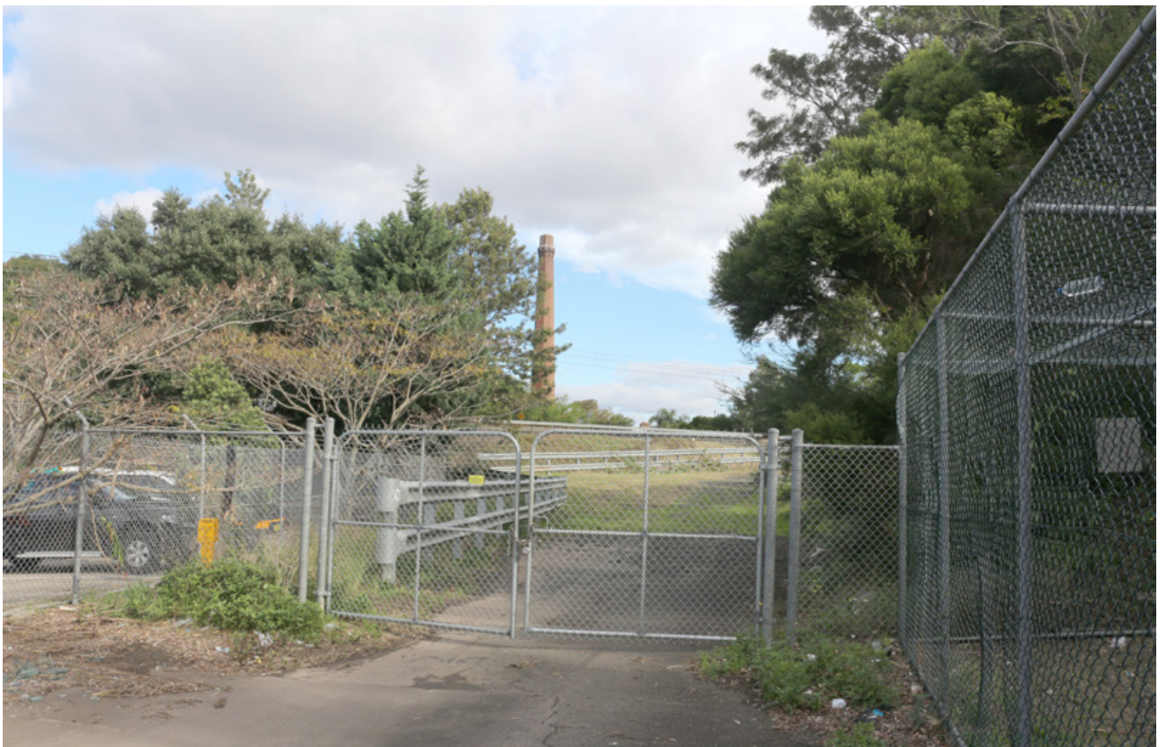
Plate 16-10 View to sewage pumping station 271 chimney stack from Fraser Park
