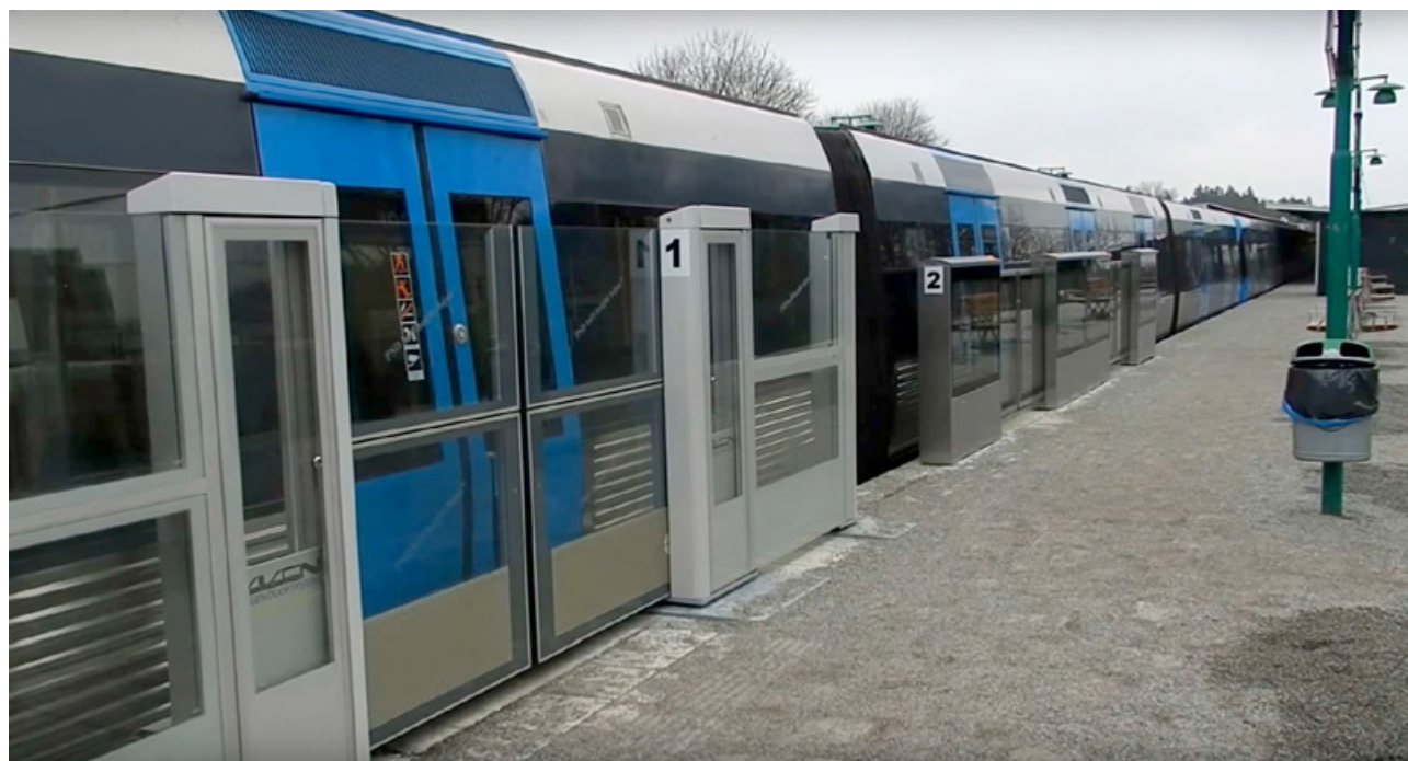
Platform Screen door at Åkeshov station Stockholm tunnelbana 2015
