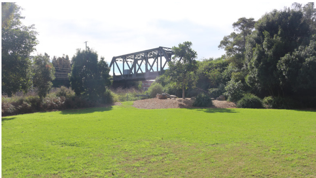
Plate 16-7 Goods Line pratt truss bridge
