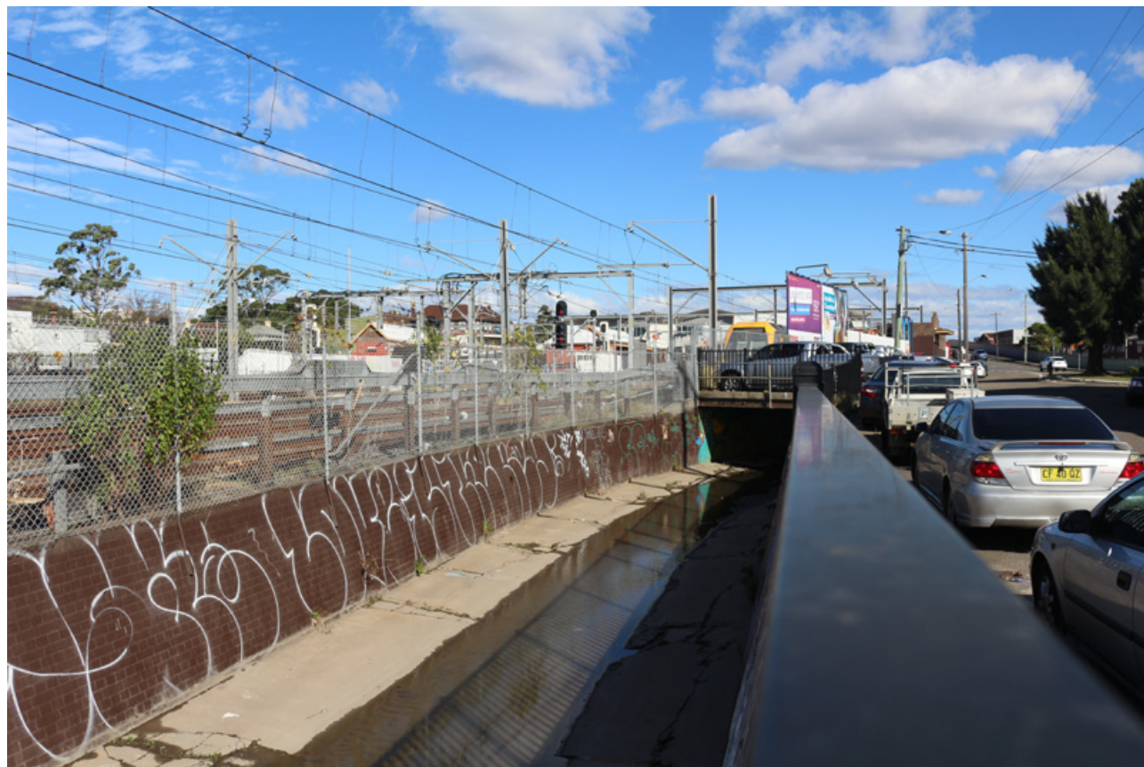
Plate 16-5 Open drain running between Railway Parade and the rail corridor near Sydenham Station
