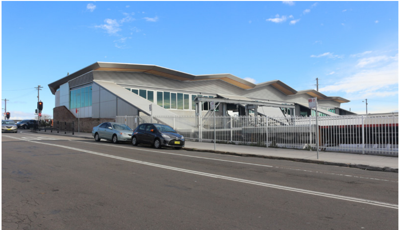
Plate 16-1 View of Sydenham Station south-west from Burrows Avenue
