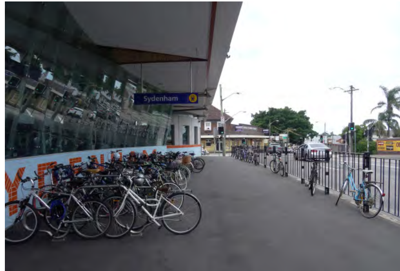
Sydenham Station entry, Gleeson Avenue Source: COX/HASELL
