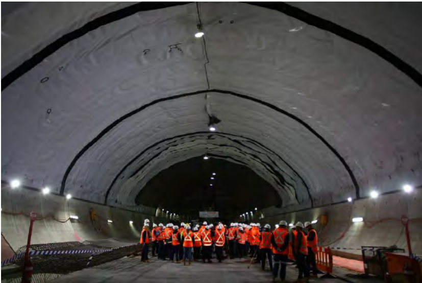
Construction of Sydney Metro Northwest. Source: TfNSW
