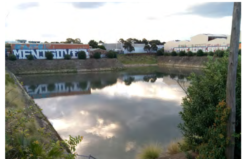
Sydenham Stormwater Storage Pit Source: COX/HASELL
