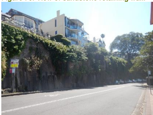
Figure 76: View of sandstone retaining wall.
