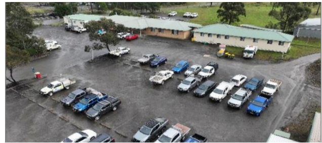
Plate ES-2 SMC Office and Carpark Area Available for Use for the Project
