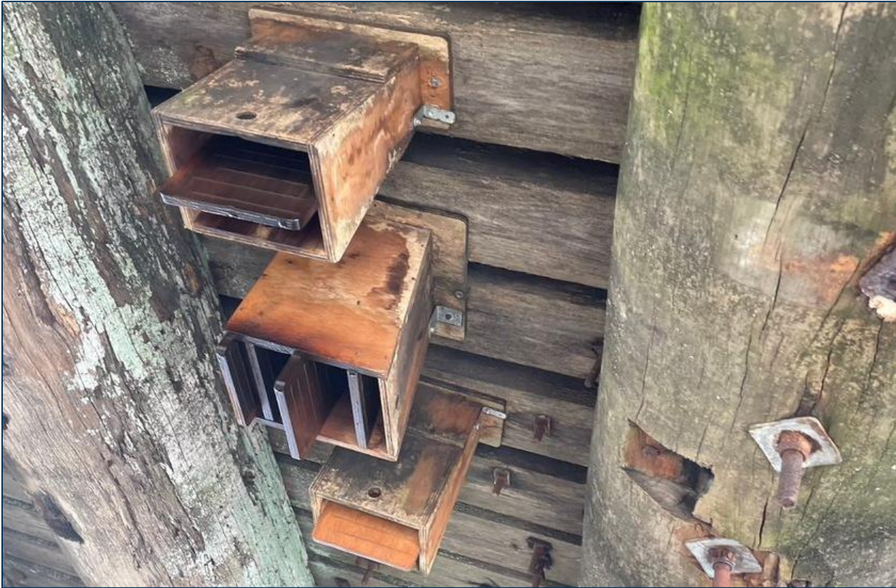
Figure 6-3 Example of a four-chamber, cave-style microbat box installed under a structure
