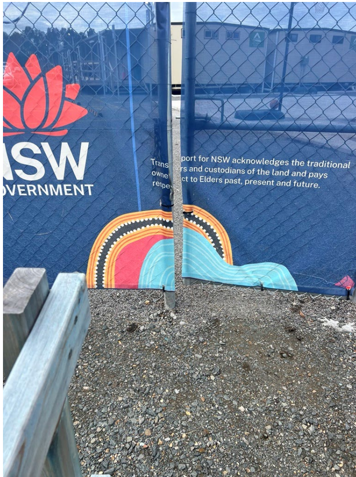
Photo 10: Boundary screening around AS5 in accordance with Condition A21
