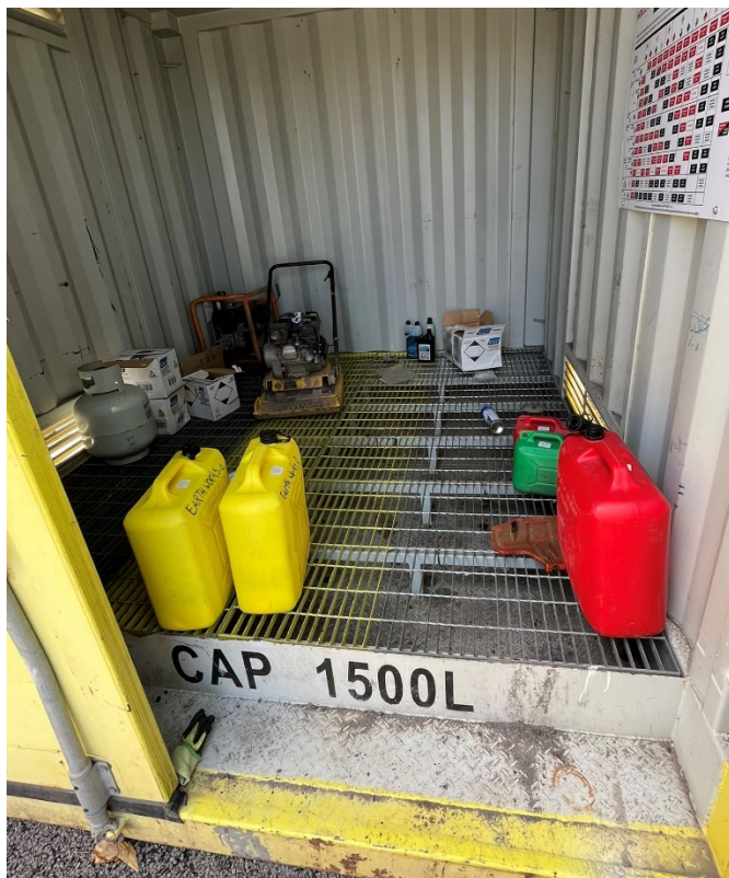
Photo 8: Fuels and chemicals appropriately stored in bunded container, JHGJV site compound BH2T
