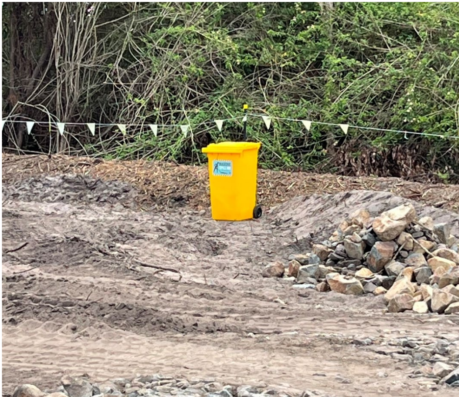
Photo 14: Spill kit at Windeyers Creek work site
