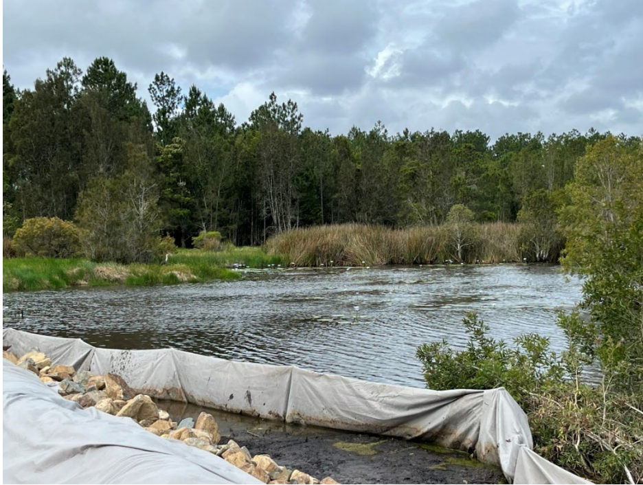
Photo 13: Geofabric curtain adjacent to temporary crossing of Windeyers Creek to prevent mobilisation of sediment into creek. Note clean rock used in crossing construction
