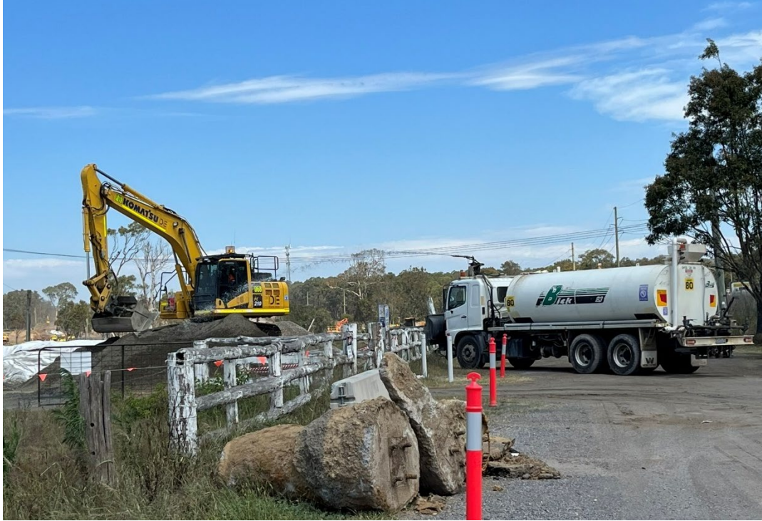
Photo 5: Water truck spraying aggregate stockpile at Gate 3 – BH2T
