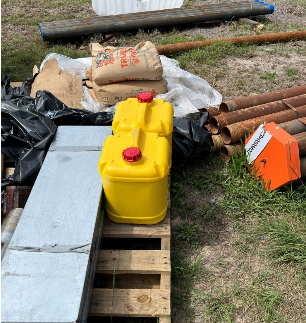
Photo 17: Containers of chemicals not placed in a bund, HBB
