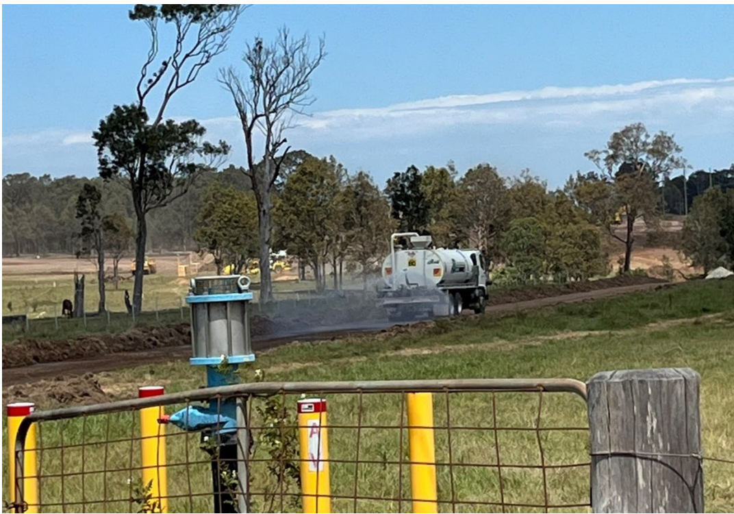
Photo 4: Water truck in use on access track to AS3 – BH2T
