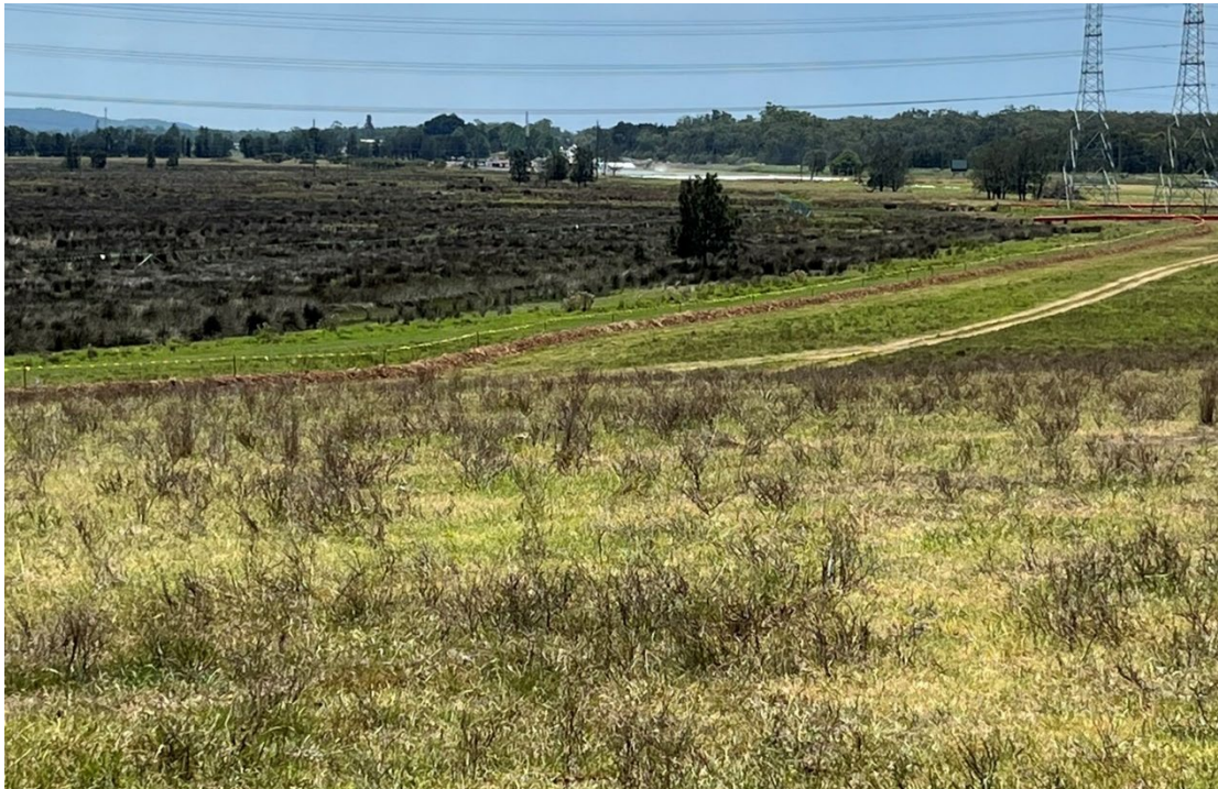
Photo 6: Mulch bund and clearing and project boundary flagging north of Cut 15 – BH2T
