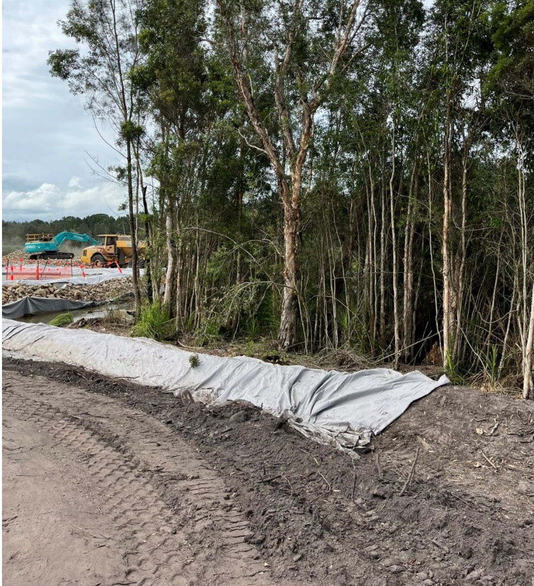
Photo 12: Substantial geofabric-covered bund installed adjacent to paperbarks near temporary waterway crossing at Windeyers Creek to prevent mobilisation of sediment
