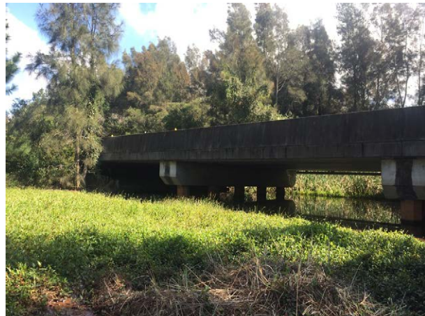
Photograph 37: Windeyers Creek bridge
