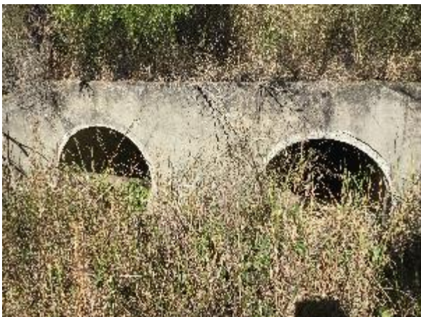
Photograph 40: Double 1200 mm culvert under the northern end of Lenaghans Drive
