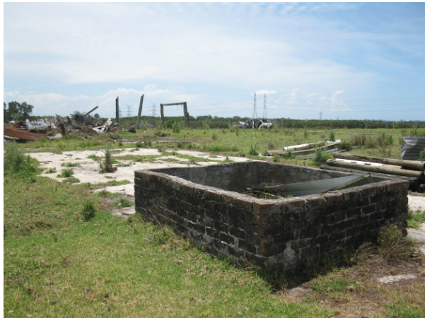
Figure 4-11 Brick tank, facing east, 15 December 2015
