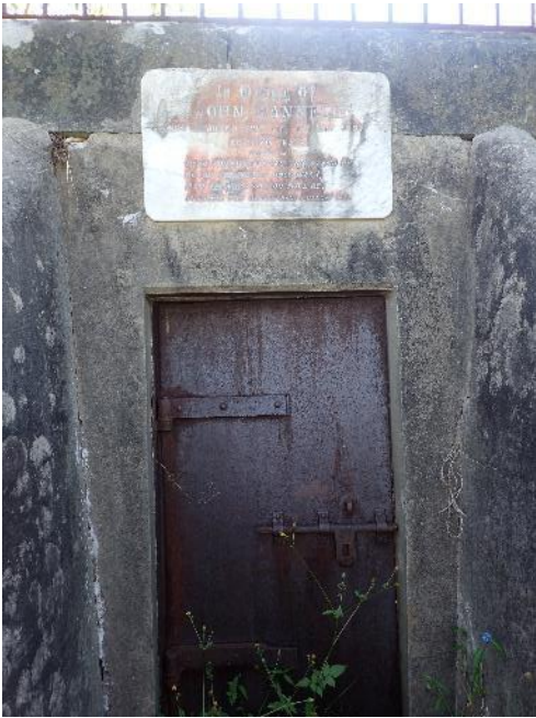
Figure 5-2 Front door of the vault
