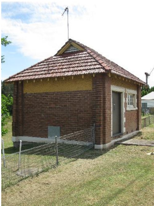
Figure 5-48 The Tarro Substation, facing southwest
