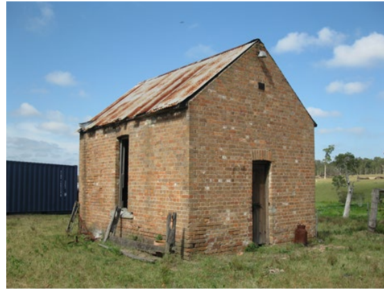
Figure 5-22 Brick store (Site 1), facing west
