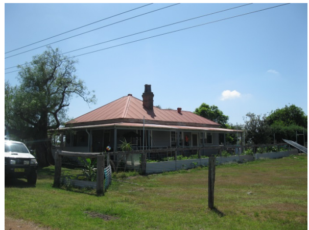
Figure 5-28 Site 2 weatherboard house, facing east
