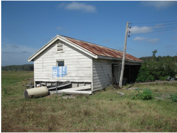
Figure 5-25 Weatherboard and cement sheeting shed (Site 1), facing west
