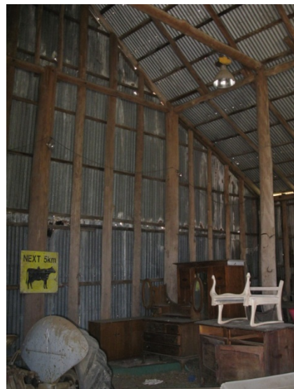
Figure 5-24 Inside of corrugated iron shed (Site 1), facing southwest
