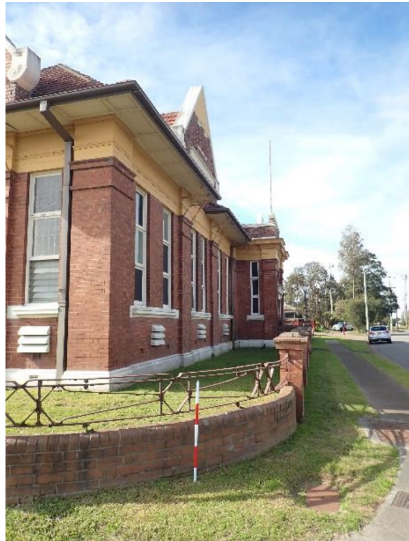
Figure 5-52 The Pumping Station, facing northeast.
