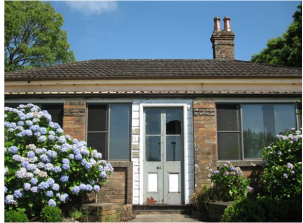
Figure 5-16 South-eastern section of brick house (Site 1), facing north
