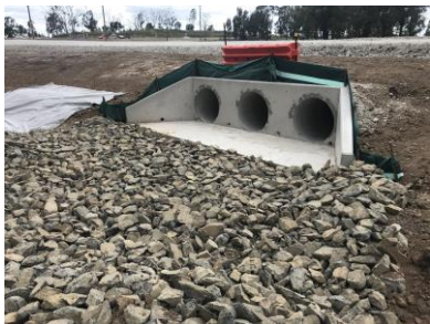
Checks have been placed in the drains at the toe of the batters
