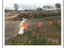
Stockpiled material has been compacted and sprayed with soil binder. The lower section has had a good dose of soil binder applied to it. Refer photo below:
