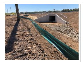
Hydro-mulch all of the areas that have not been hyrdo-mulched yet (ie above the culvert headwall and drain to the north of the inlet.
