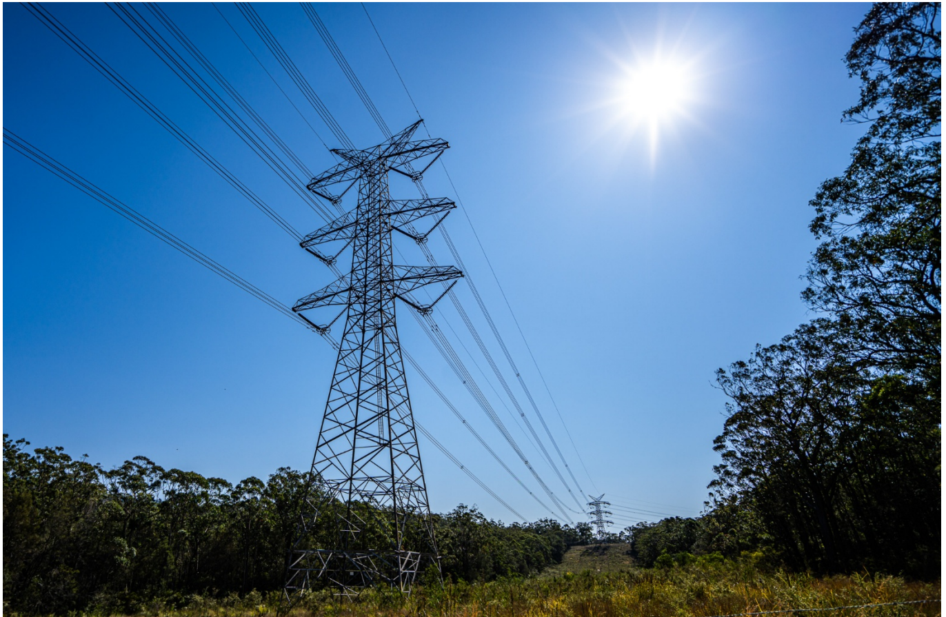
Image A-1 Example 500 kV double circuit transmission line and towers (Eraring to Kemps Creek)
