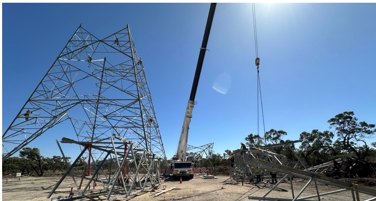
Image A-2 Example 500 kV transmission line tower being assembled for Project EnergyConnect
