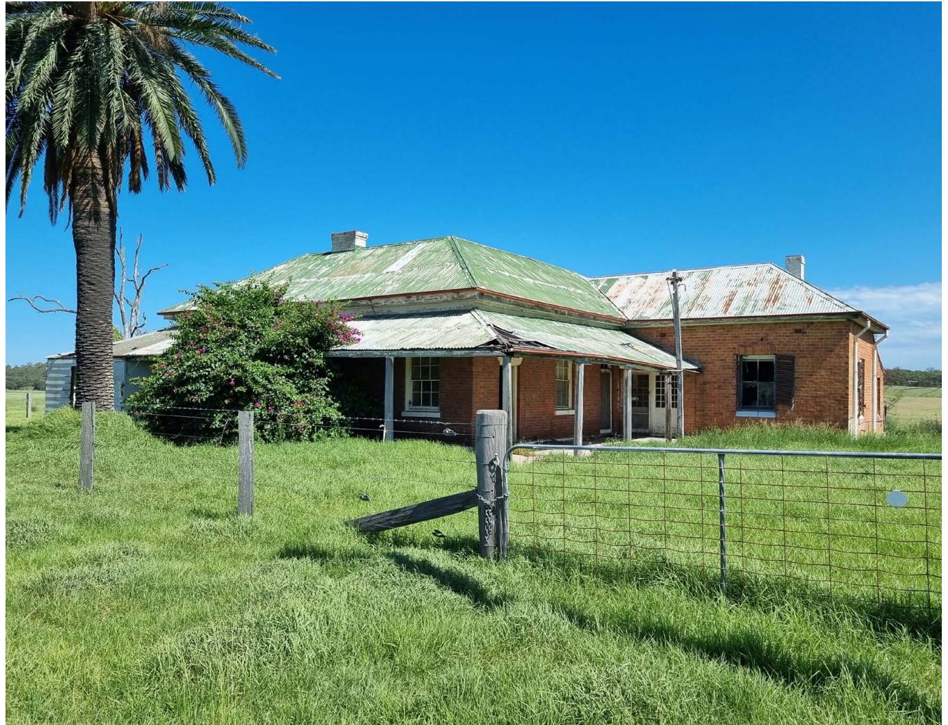
Historic heritage surveys – ‘Stafford’ homestead, Warkworth
