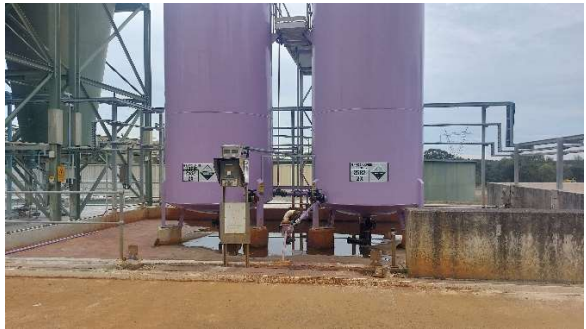
Photo 5. Storage of chemicals used in flocculant processes
