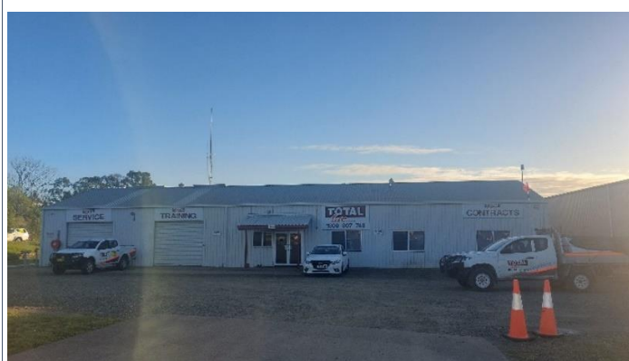
Photo 1. Total Fire – assumed to store minor amounts of firefighting foam
