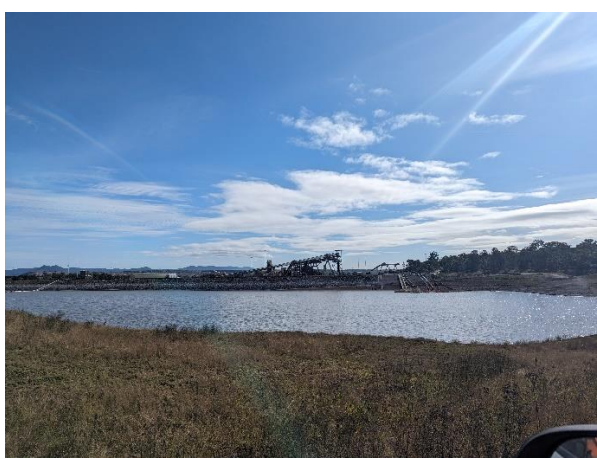
Photo 1. Dam – assumed to support the coal handling plant
