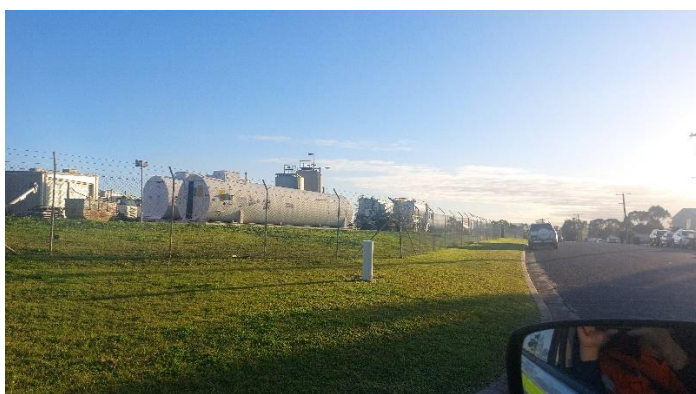
Photo 4. Orica fuel depot – above ground storage tanks and fuel infrastructure
