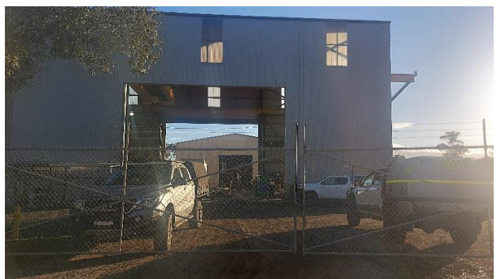
Photo 12. Monadelphous – engineering company. Mining and mechanical infrastructure across the site
