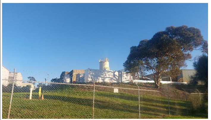
Photo 8. Enaex – ASTs and fuel infrastructure
