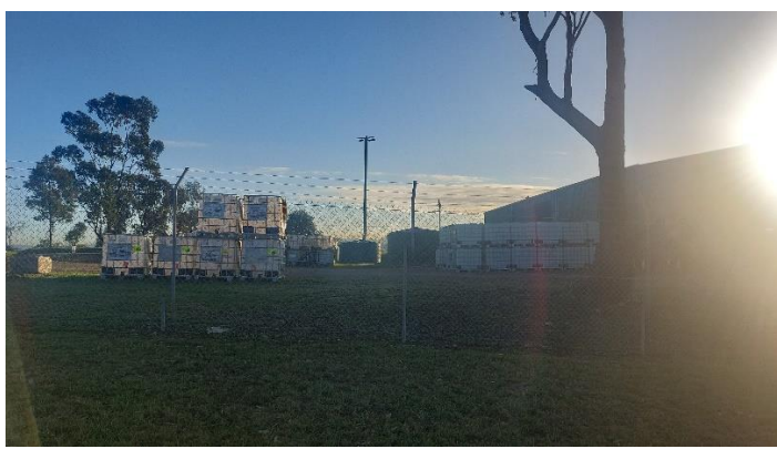
Photo 7. Enaex – ASTs, containers, IBCs and drums observed on site
