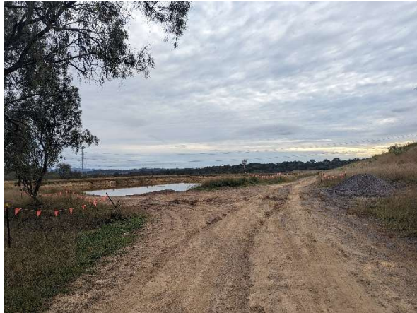
Photo 3. Multiple dams present on site
