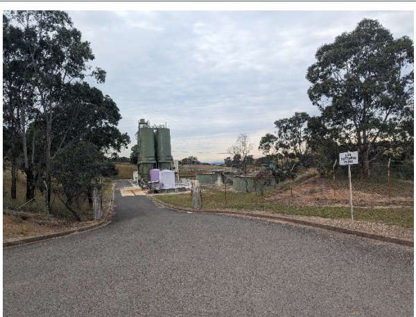
Photo 1. Lime softening plant
