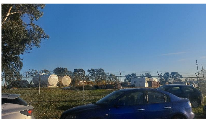
Photo 6. Enaex – ASTs, containers, IBCs and drums observed on site
