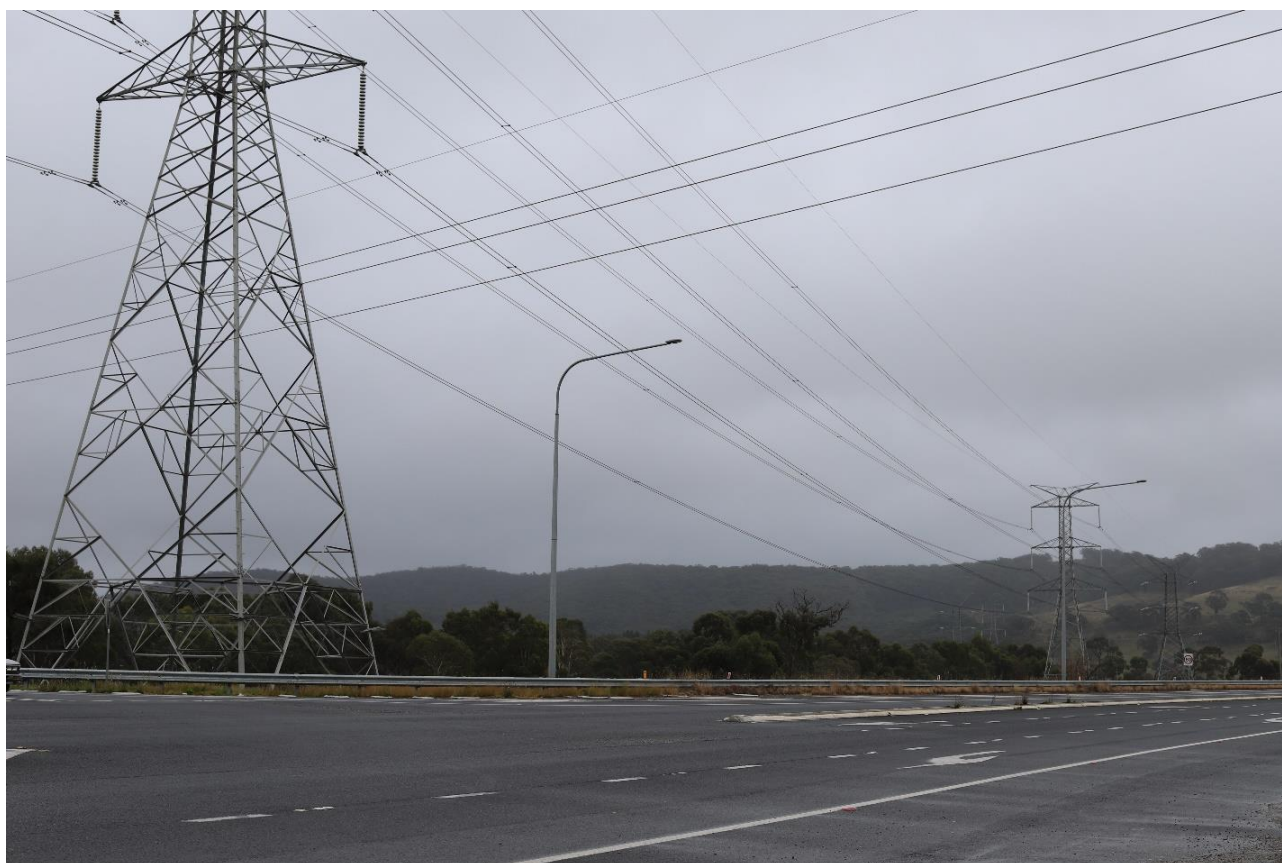
Figure 6.8 View at VP09 along Castlereagh Highway west of Main Street including existing transmission infrastructure
