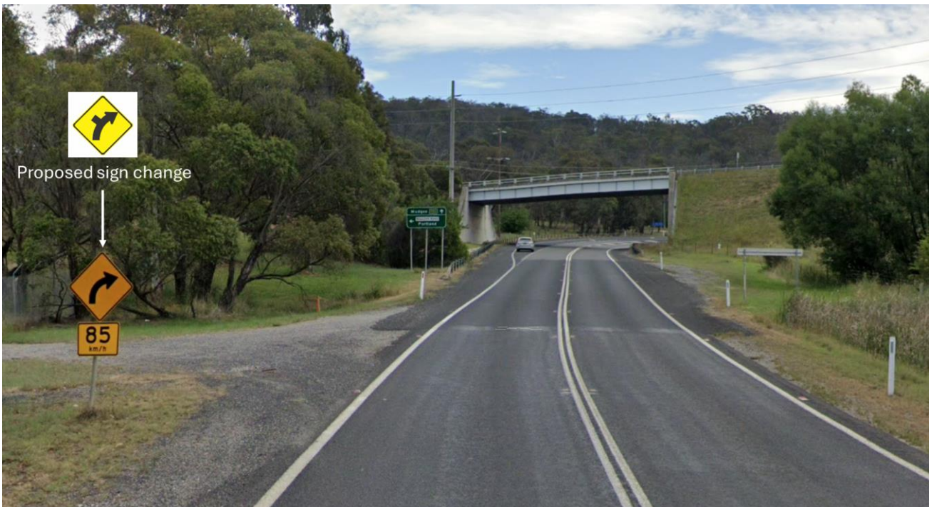
Figure 4.21 Available and required sight distance at Boulder Road / Mount Piper Power Station Access
