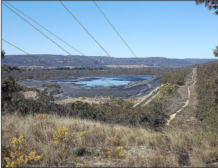
View southeast within the project area towards Wallerawang.
