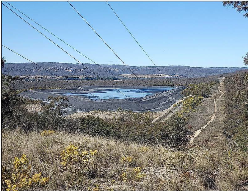
View east overlooking the existing Mount Piper to Wallerawang transmission line and easement.
