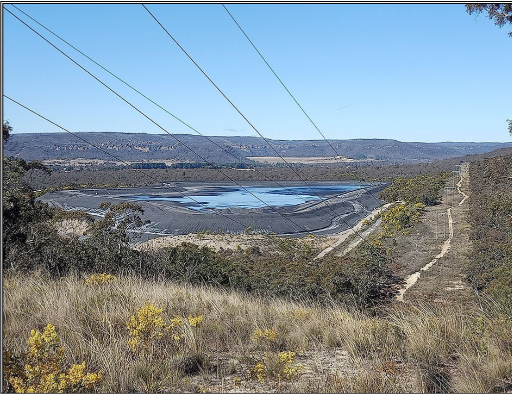
View southeast along existing transmission line easement within the project footprint.
