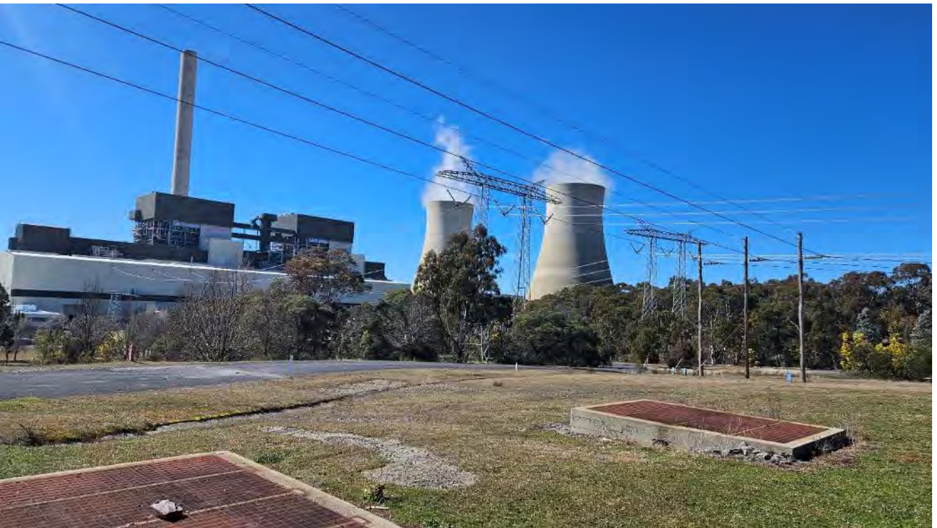
Figure 15 View of the Mount Piper Power Station from Mount Piper 330 kV/500 kV substation
