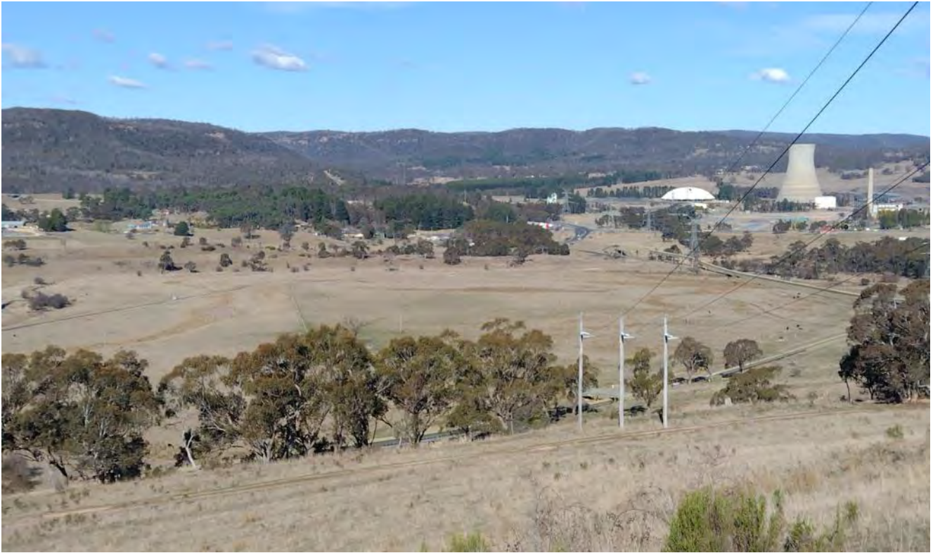
Figure 16 View from the existing 132 kV Line 94E easement to adjacent agricultural land, looking towards the Castlereagh Highway and the former Wallerawang Power Station.
