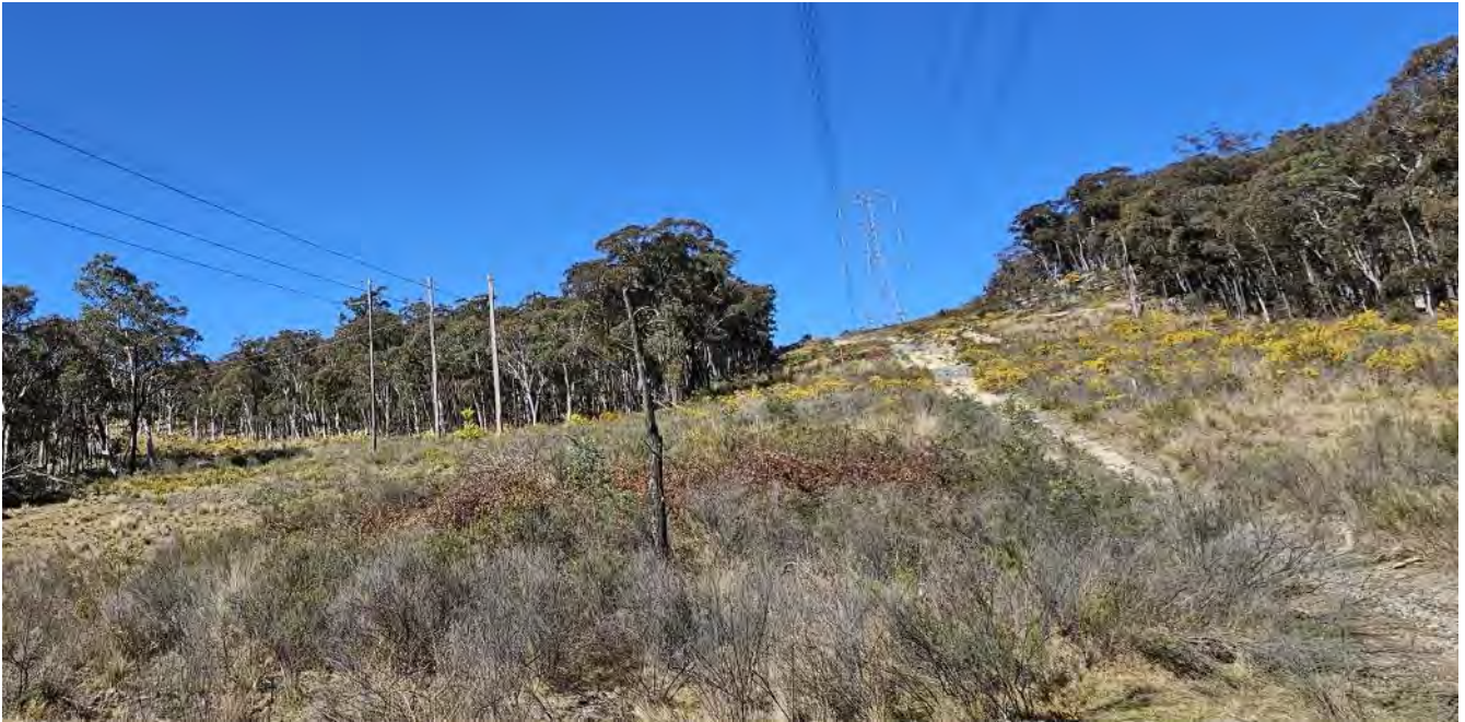
Figure 3 Existing infrastructure in the easements near Mount Piper: timber poles supporting the 132 kV Line 94E (left) and steel transmission structures supporting the 330 kV Line 70/71 (right).
