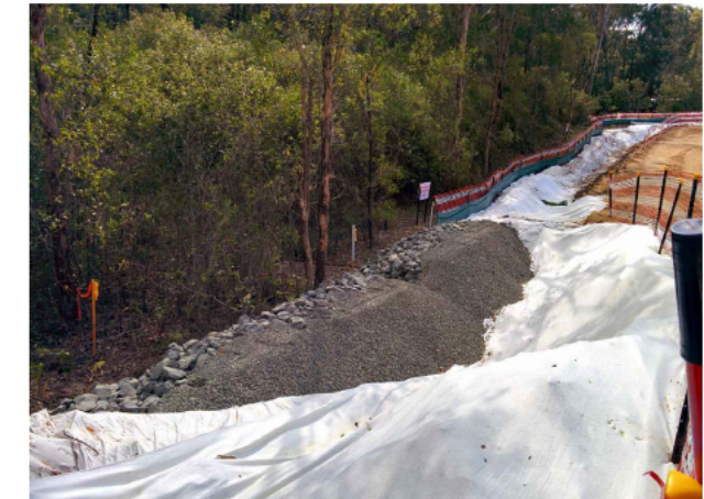
PHOTO 3 - EXAMPLE OF ROCK FILTER DAM AND SUMP
