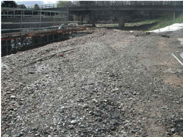
PHOTO 6 - EXAMPLE OF A PILING PLATFORM STABILISED SURFACE
