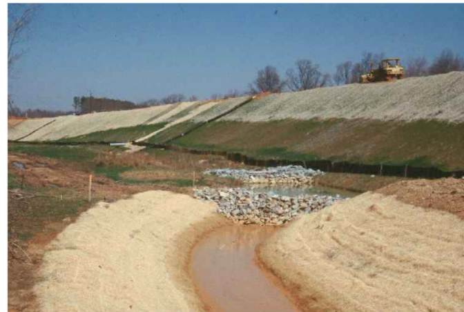
PHOTO 2 - PROGRESSIVE STABILISATION OF BATTERS AS WORKS PROGRESS
