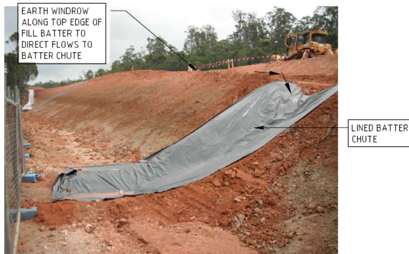
PHOTO 4 - EXAMPLE OF BATTER CHUTE
