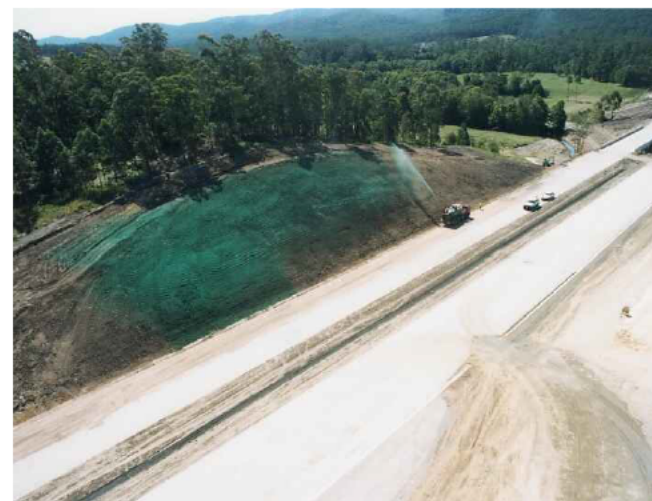
PHOTO 5 - TEMPORARY STABILISATION OF BATTERS WITH POLYMER
