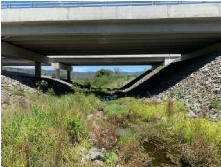
Photo 2 Frazer Creek Rehabilitation works and bridge scour protection
