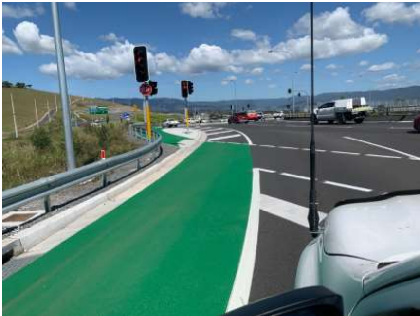
Photo 7 Completed Road and Operational Signage
