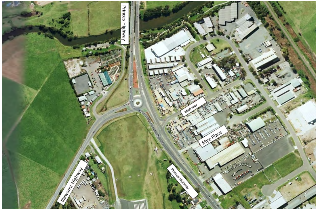
Figure 4-13 Existing Princes Highway / Illawarra Highway Intersection
