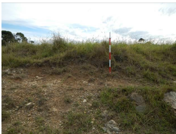
Plate 29: Survey Unit 7 – erosion at confluence of Frazers Creek and its tributary, view to NE.
