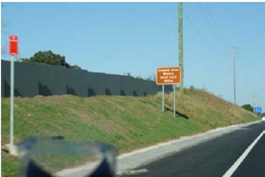
Plate 4-3: Precedent of Noise Walls
