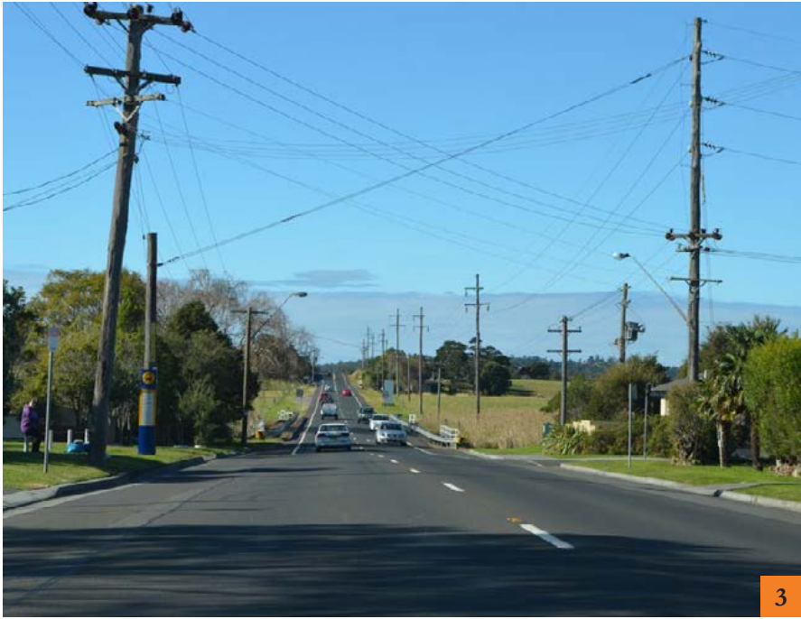
Plate 2-3: View along Tongarra Road heading towards Albion Park Rail
