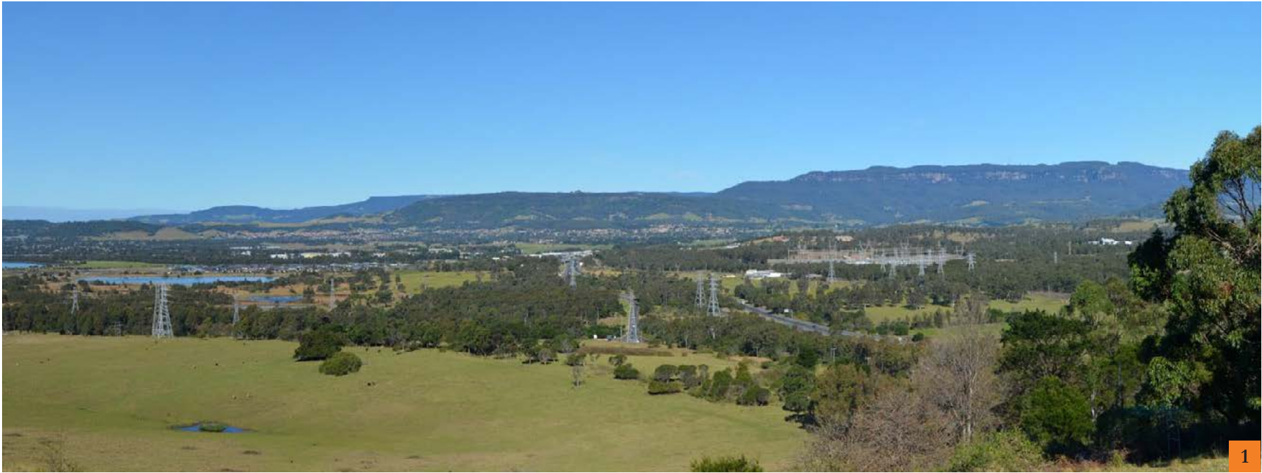
Plate 2-1: View from the Dapto hills looking south
