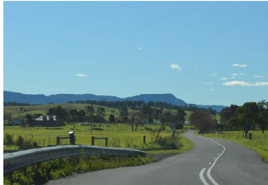
Plate 2-18: Calderwood Road heading north in Calderwood
