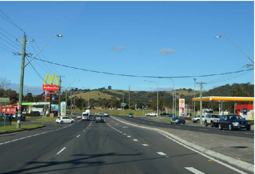
Plate 2-8: Highway commercial activity in Albion Park Rail along Princes Highway looking south.
