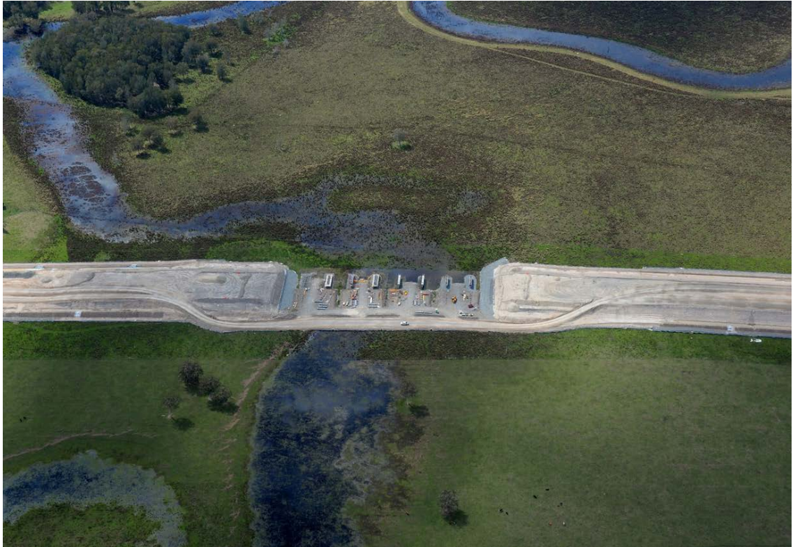
Figure 5-28 Example temporary side track at a bridge for small creek crossing – constructed and operational
