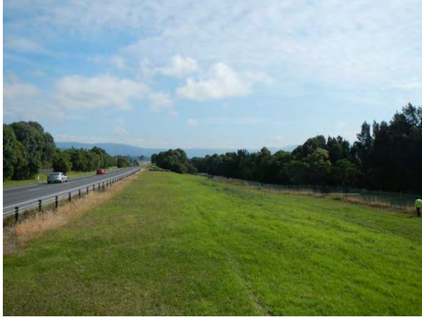
Plate 19: Survey Unit 6 – massive embankment and road bund along northern edge of East West Link, view to W.
