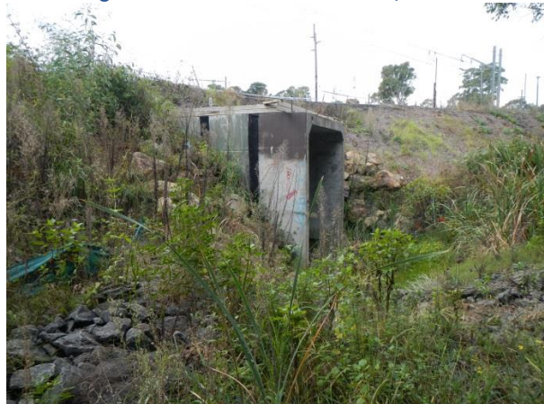
Plate 6: Survey Unit 2 – railway embankment and drainage channel/drain in the north, view to SE.
