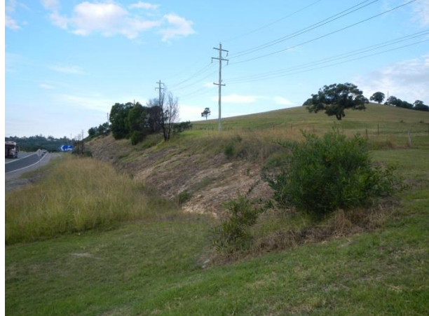
Plate 22: Survey Unit 6 – cutting through slope and crest landform to south of East West Link, view to E.
