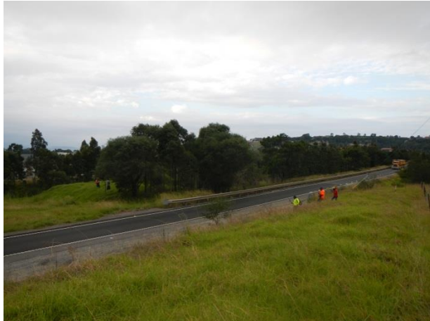
Plate 24: Survey Unit 6 – disturbed island between the branches of the East West Link, view to NE.
