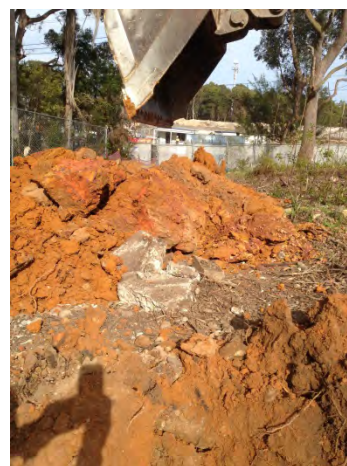
Photo 8 – Former concrete slab at TP60. Photo looking southwest towards site office
