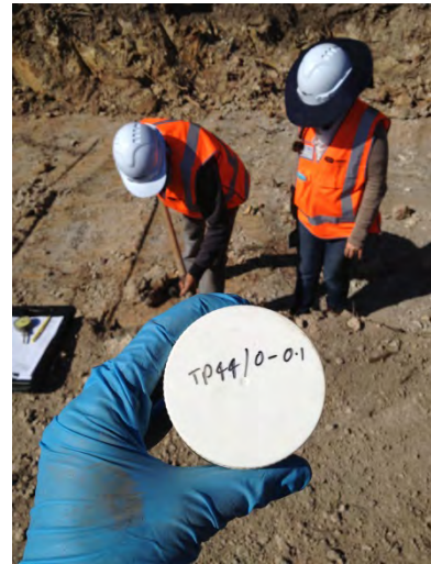
Photo 18 – TP44 – The open service trench along the southern site boundary was utilised for sampling at this location
