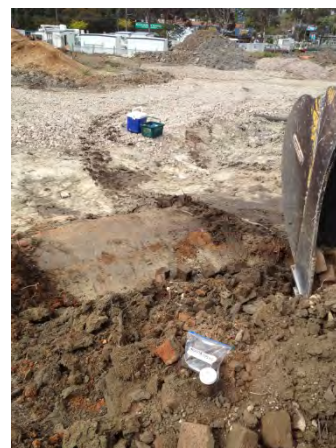
Photo 6 – TP29A – bricks and topsoil encountered in former garden. Photo looking southeast towards site office and Warringah Road
