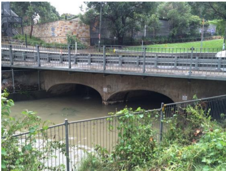
Plate 11 Culvert and footway from southern bank
