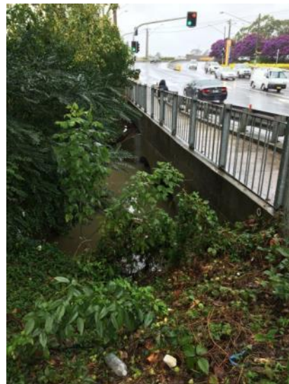
Plate 12 Downstream side of culvert from northern bank
