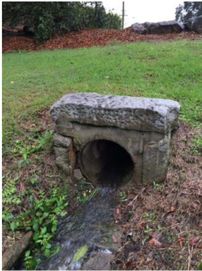
Plate 8 Sandstone and concrete drain
