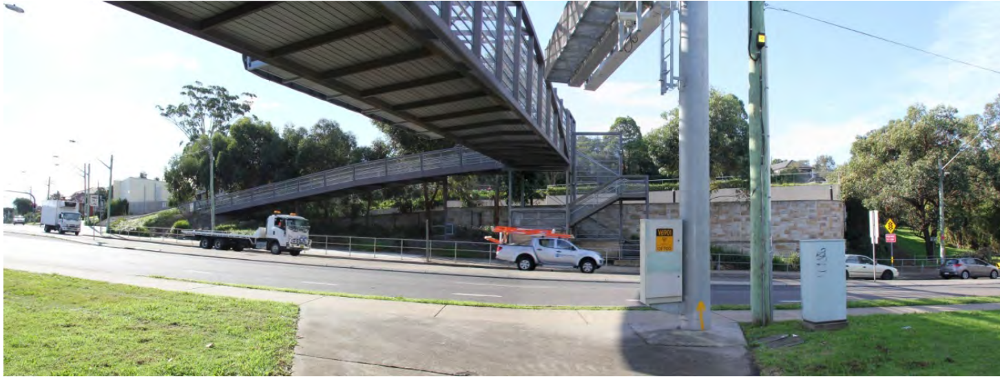
Figure 4-26 View east from the exit of the pedestrian overpass to the Bexley East site area (Bexley Road East construction compound), which lies beyond the sandstone wall
