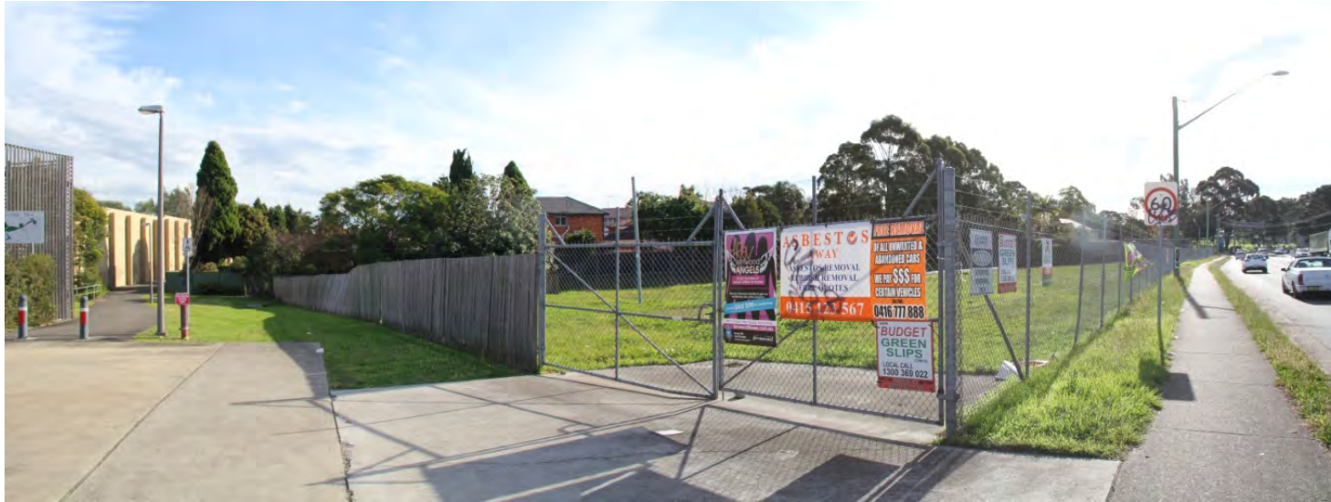
Figure 4-24 Bexley Road surface works site area: Bexley north (Bexley Road North construction compound), with the entry to the M5 Linear Park to the left of frame and Bexley Road to right of frame
