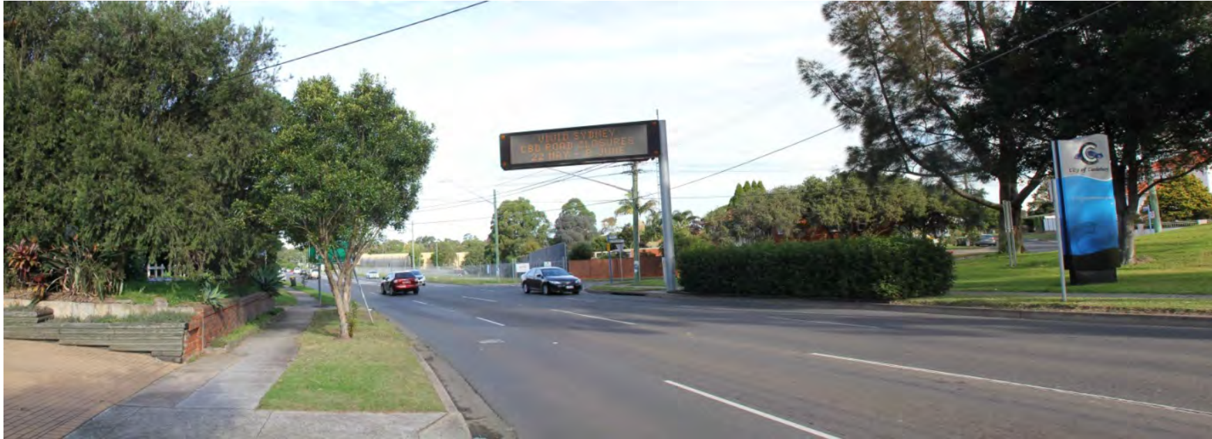
Figure 6-15 The view south along Bexley Road from just north of Poole Street, towards the Bexley Road North construction compound
