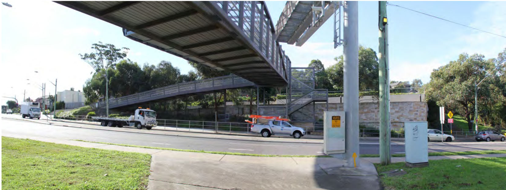
Figure 6-23 View east from the pedestrian exit to the Bexley Road overpass back to the Bexley Road East construction compound. Note the house seen above the stone wall to the right of frame, which is representative of homes on Johnston Street that overlook the compound site
