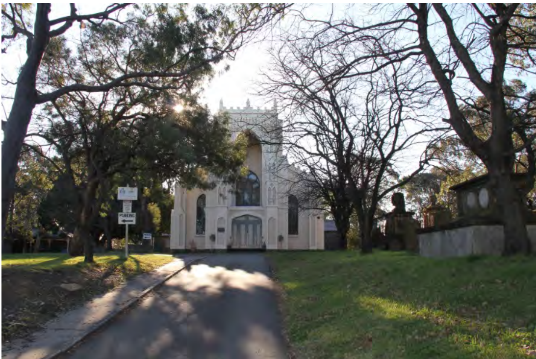
Figure 6-32 The heritage listed St Peters Anglican Church, which sits on a localised hill on the northern side of the Princes Highway, but set back from the highway amongst a park setting of turf and trees.
