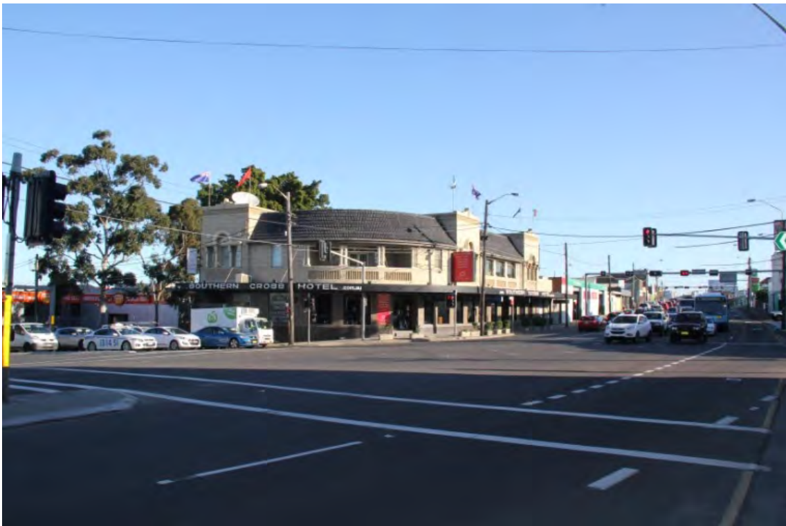
Figure 6-29 The Southern Cross Hotel on the corner of the Princes Highway and Canal Road
