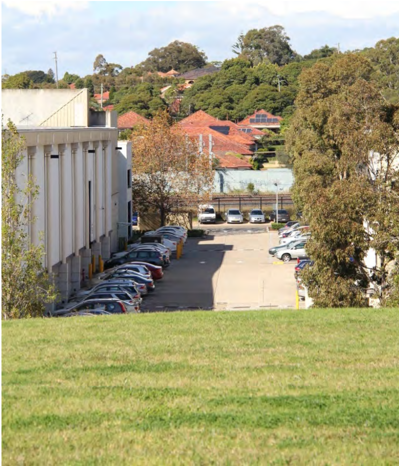
Figure 6-10 View between large scale industrial complexes fronting Vanessa Street, with the rail line in the middle ground and residential areas beyond
