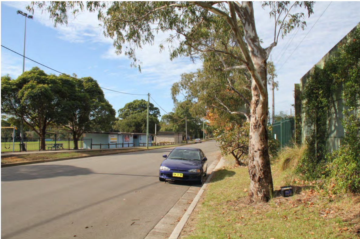
Figure 4-41 Views into and out of the rail corridor between stations are limited by noise walls and screening vegetation (to right of frame)
