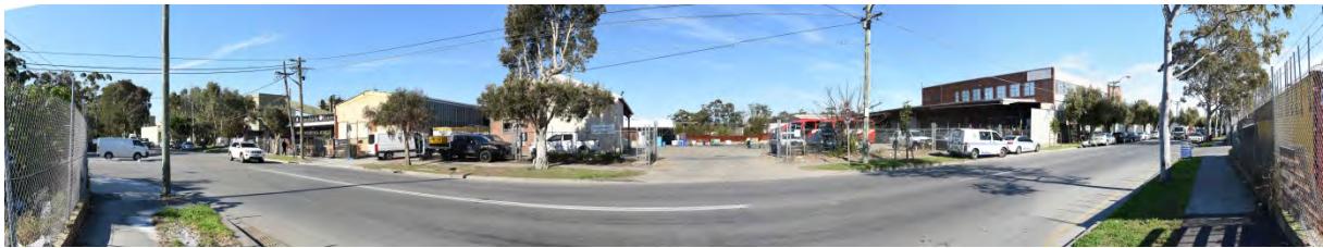
Figure 6-42 The view to the Campbell Road bridge construction compound from Burrows Road, with the Alexandra Canal in the background
