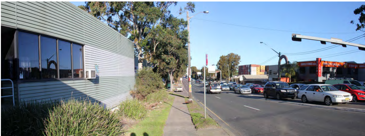
Figure 4-70 View southeast along Canal Road from the Princes Highway, showing industrial development flanking the road, and mature street trees
