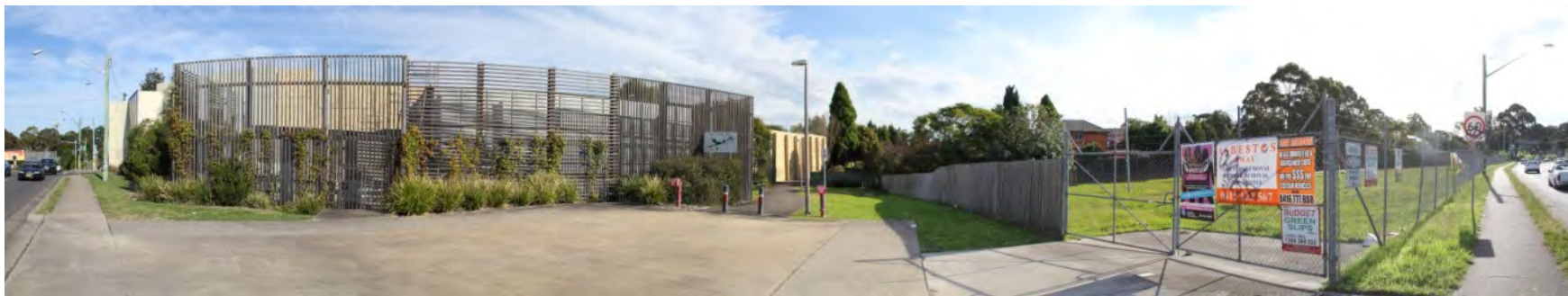
Figure 6-16 The entry to the M5 Linear Park, positioned between noise walls and infrastructure associated with the M5 East Motorway, and the Bexley Road North construction compound to right of frame
