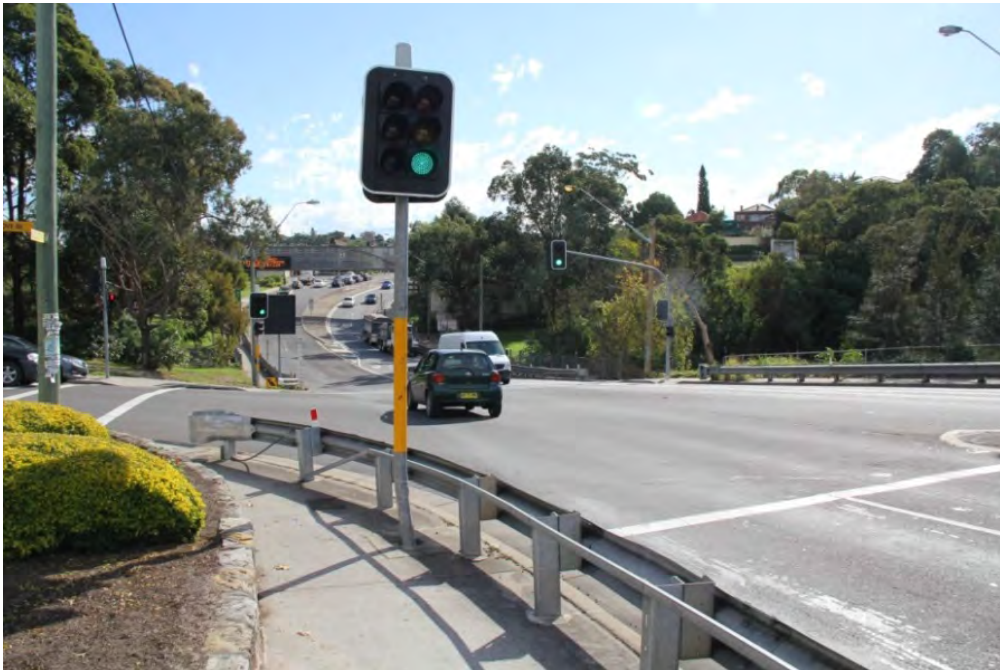
Figure 4-33 View to the Bexley East construction compound site from the intersection of Bexley Road and Kingsgrove Avenue
