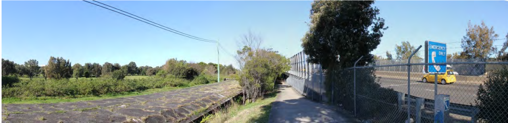
Figure 6-25 The view south-west along the Eve Street Cycleway showing the M5 East Motorway (right of frame), screening vegetation, the Western Outfall Main Sewer and the Kogarah Golf course to left of frame
