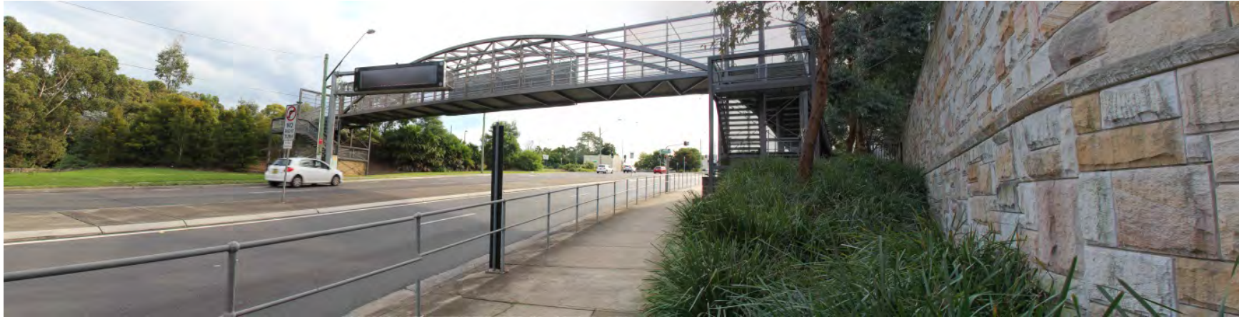
Figure 6-21 The view from Bexley Road south of the pedestrian overpass where the pedestrian path that joins Johnston Street to Bexley Road exits, looking back towards the entry of the M5 Linear Park, past the Bexley Road East construction compound situated behind the sandstone wall to the right of frame.
