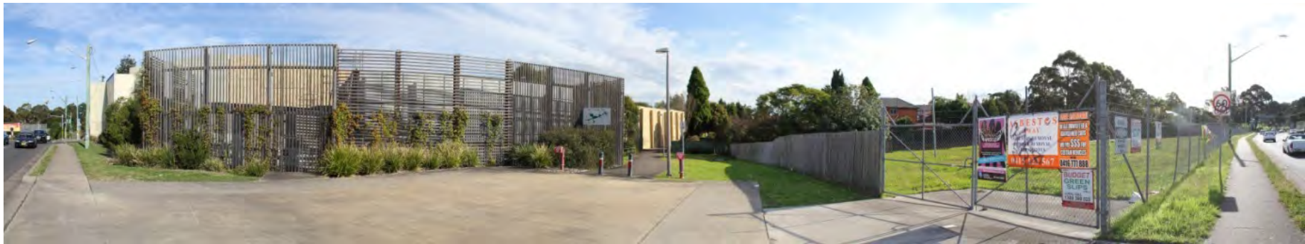
Figure 6-14 The M5 East Motorway noise walls, with the entry to the M5 Linear Park and the Bexley Road North construction compound to right of frame
