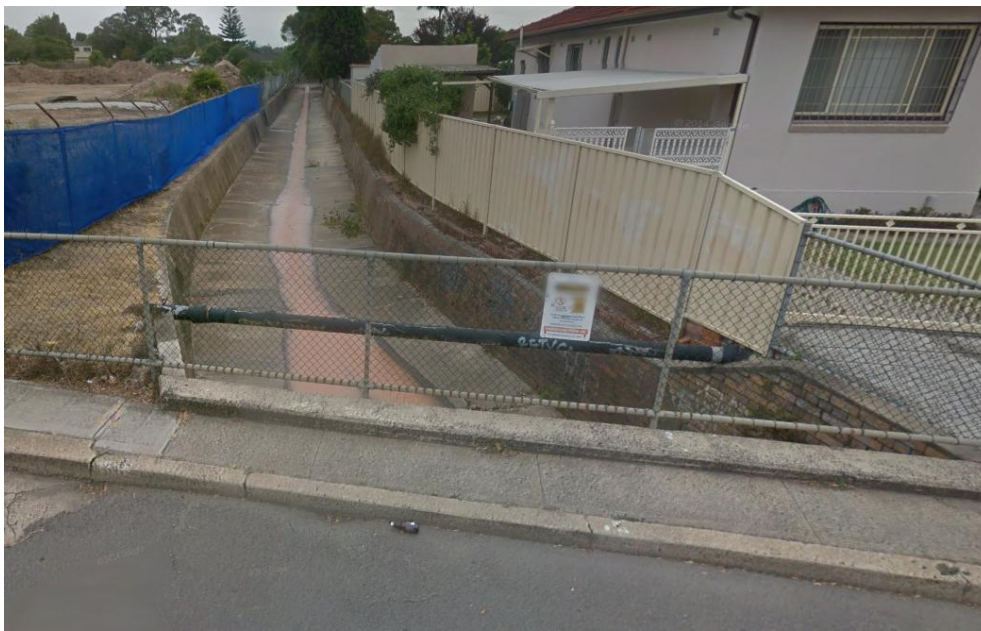
Photo 1: Stormwater channel ( on Alfred Street (looking east) (Source: Google Maps, 2016)
