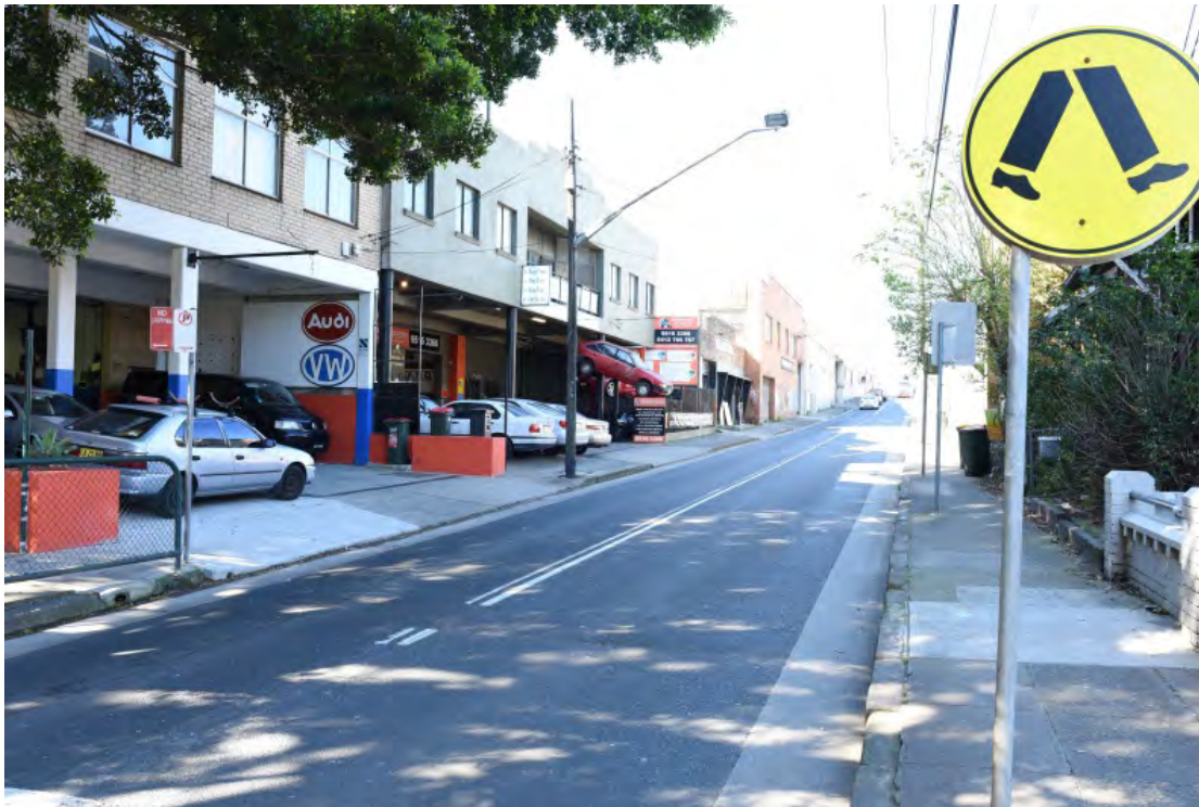
Figure 6-90 View north along Campbell Street showing industrial / commercial buildings on the north-eastern side of the road (to be retained) and residential housing on the south-western side of the road (to be removed)
