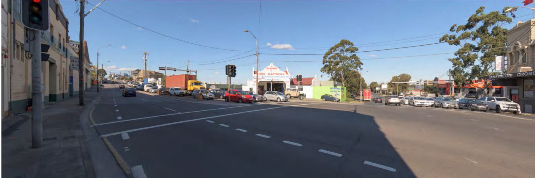
Figure 6-78 The view to the Dynamo building from the corner of Canal Road and the Princes Highway, looking south along Canal Road
