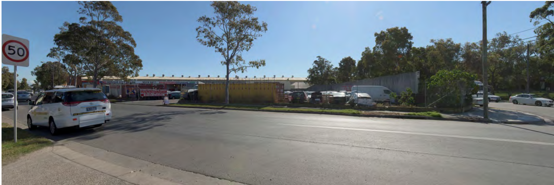
Figure 6-98 Existing view from Burrows Road to the industrial buildings on the intersection of Burrows Road and Campbell Road (seen to right of frame)
