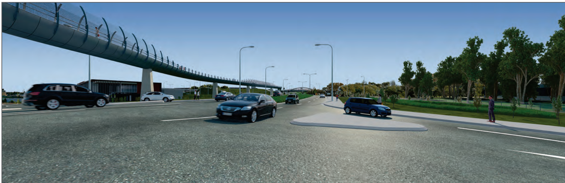
Figure 6-99 Photomontage showing the widened and realigned Campbell Road from the corner of Burrows Road, with Sydney Park to right of frame and pedestrian bridge to left of frame, at opening
