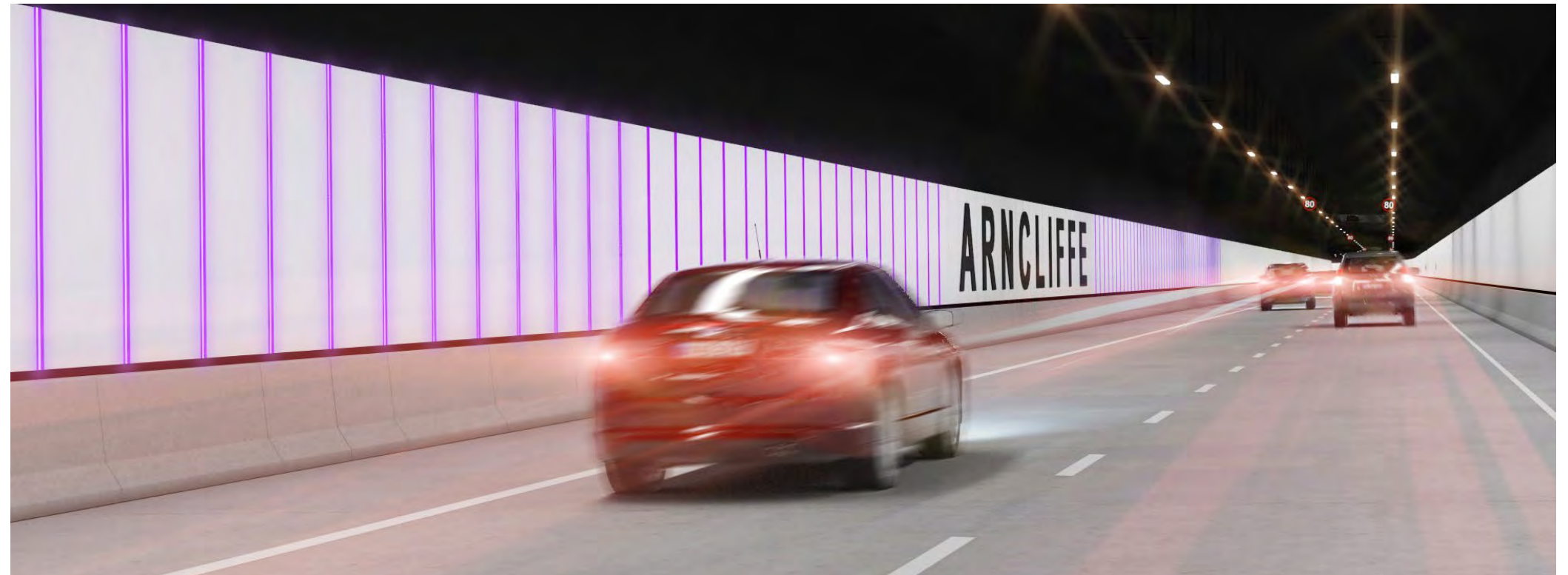
Figure 49 Visualisation of tunnel location identifier
