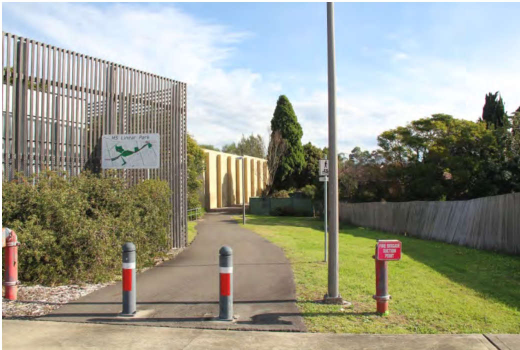
Figure 4-28 Noise and screening walls associated with the M5 East Motorway
