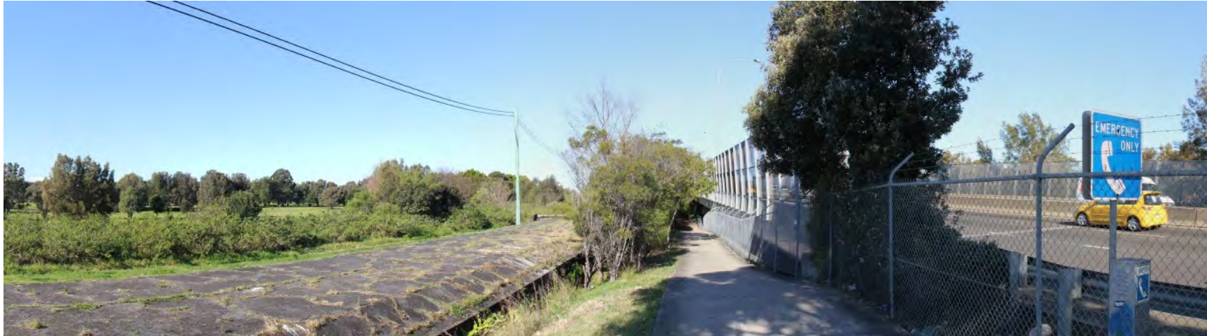
Figure 4-47 View from the Eve Street cycleway showing the relationship of the M5 East Motorway (to right of frame, screened by vegetation), the Western Outfall Main Sewer, the cycle path, and the Kogarah Golf Course (beyond the fence to the left of frame).
