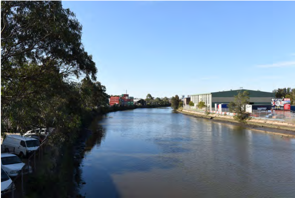
Figure 4-55 Typical view of industrial complexes flanking the Alexandra Canal (view taken from Rickettys Bridge looking north)
