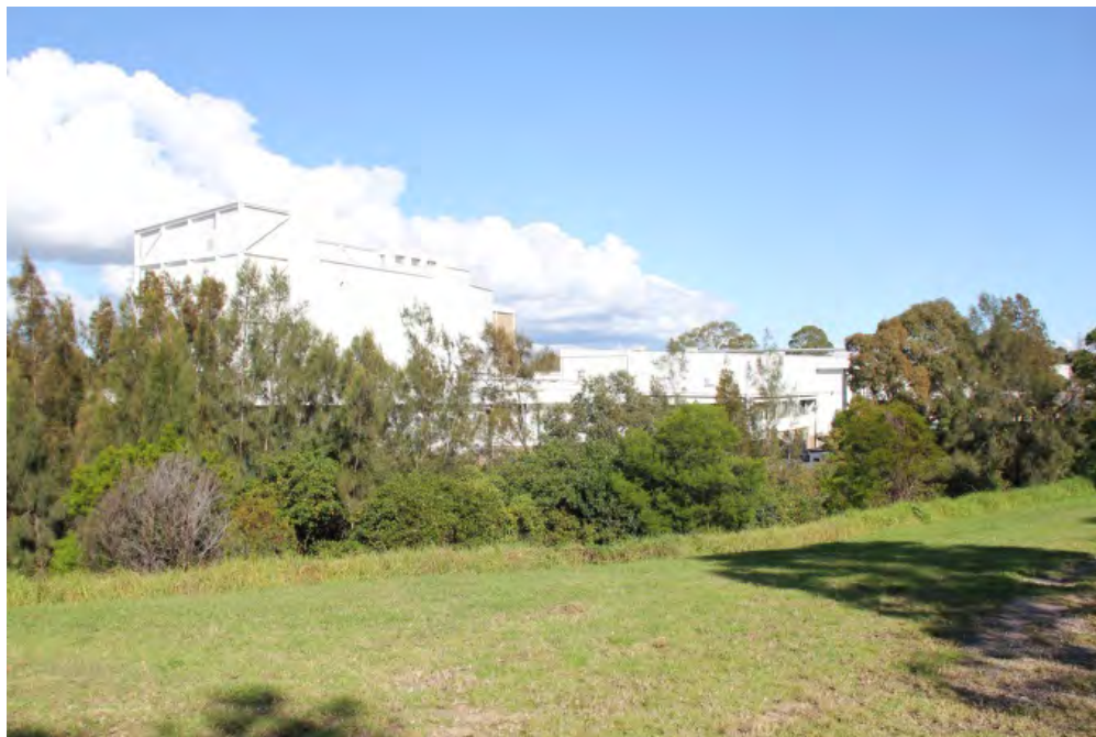
Figure 4-18 Large scale industrial complexes on the southern edge of Wolli Creek channel to the south of the M5 East Motorway
