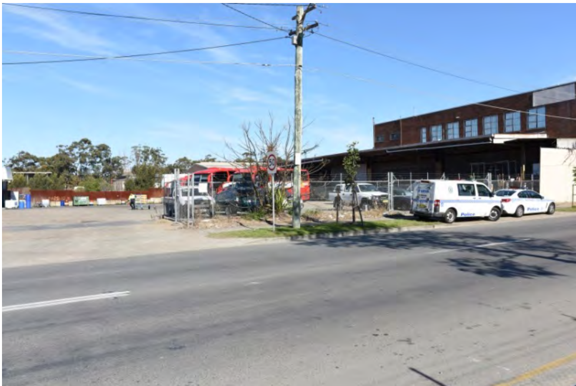
Figure 4-64 Glimpse views can be seen between industrial buildings to the Alexandra Canal
