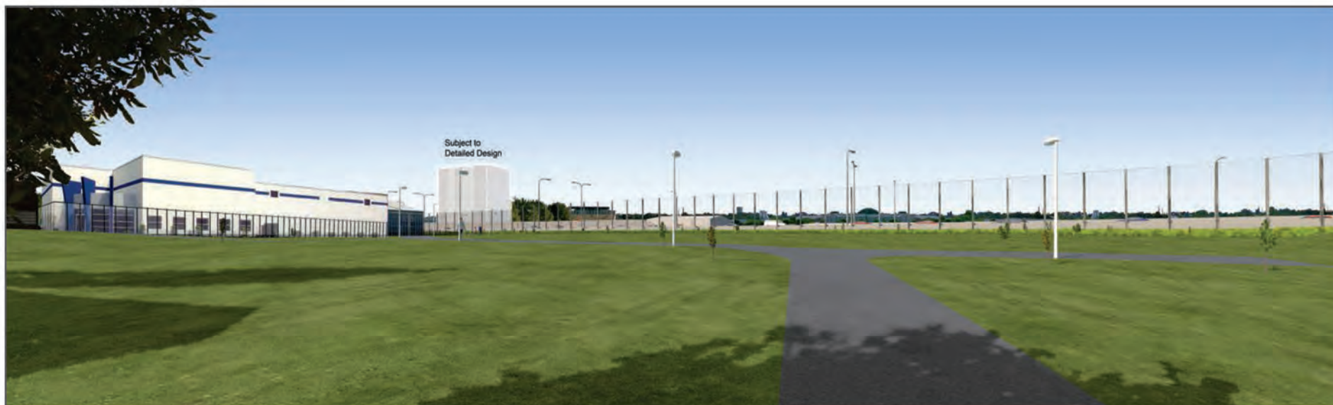
View to south - across Beverly Grove Park to New M5 motorway - project completion
