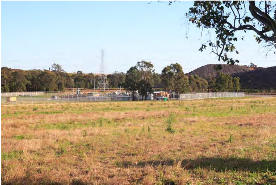
Plate 6-1 Photo of the facility
