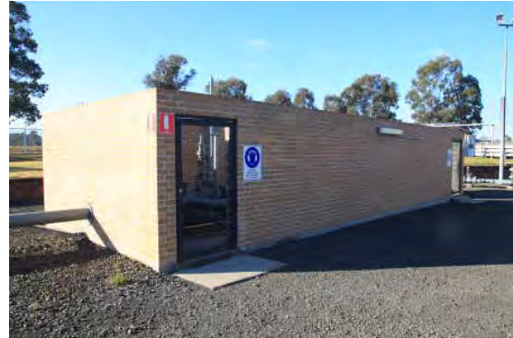
Plate 1-2 Regulator gas for delivery to the Smithfield Lateral (inside masonry enclosure)
