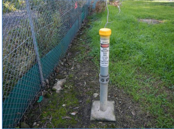
Figure 7: View to the East, signage showing presence of subsurface infrastructure.
