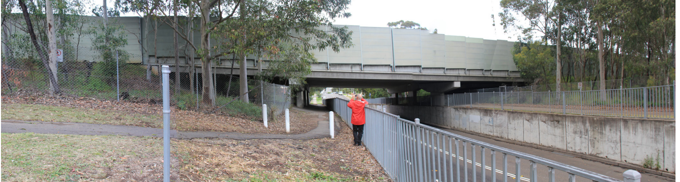
Figure 67 Panorama showing existing M5 Motorway bridge spanning Penshurst Road
