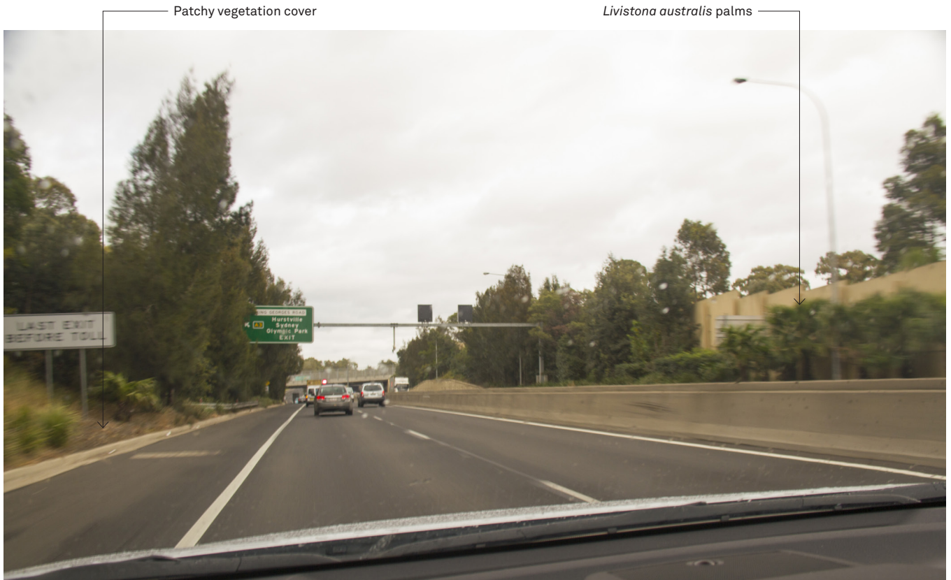
Figure 59 Existing view from passenger seat of vehicle travelling west on the M5 Motorway, towards Cooalongatta Road bridge
