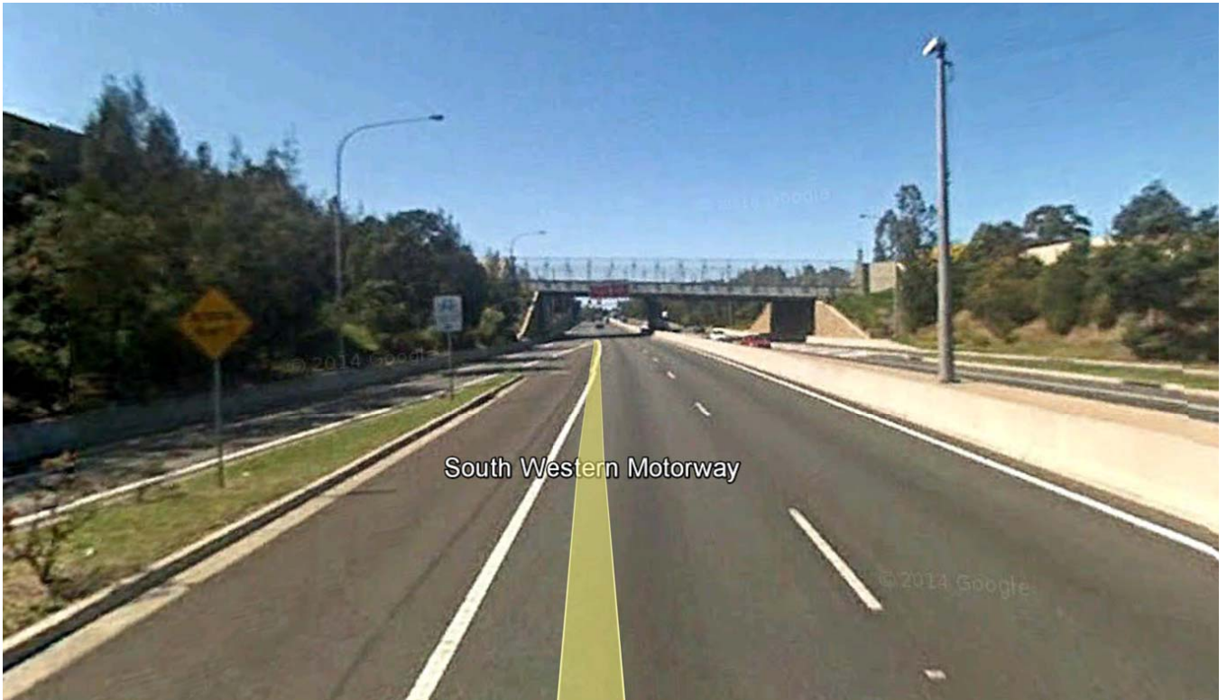
Figure 63 View of existing Motorway looking east, travelling towards Cooloongatta Road bridge (Source: Google Earth Street View)
