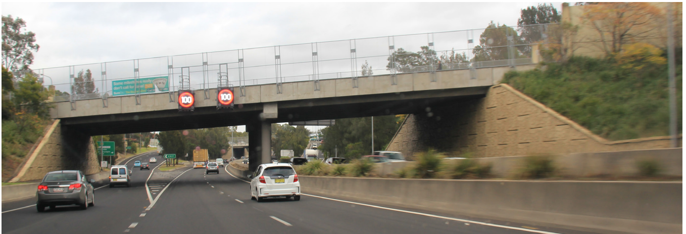
Figure 17 Reinforced earth wall details associated with existing bridges are not well coordinated with other urban design elements such as the adjacent bridge deck.
