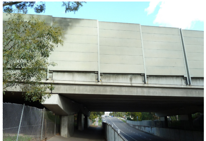
Figure 16 To the west of the King Georges Road Interchange the walls consist of long, narrow aerated concrete panels.
