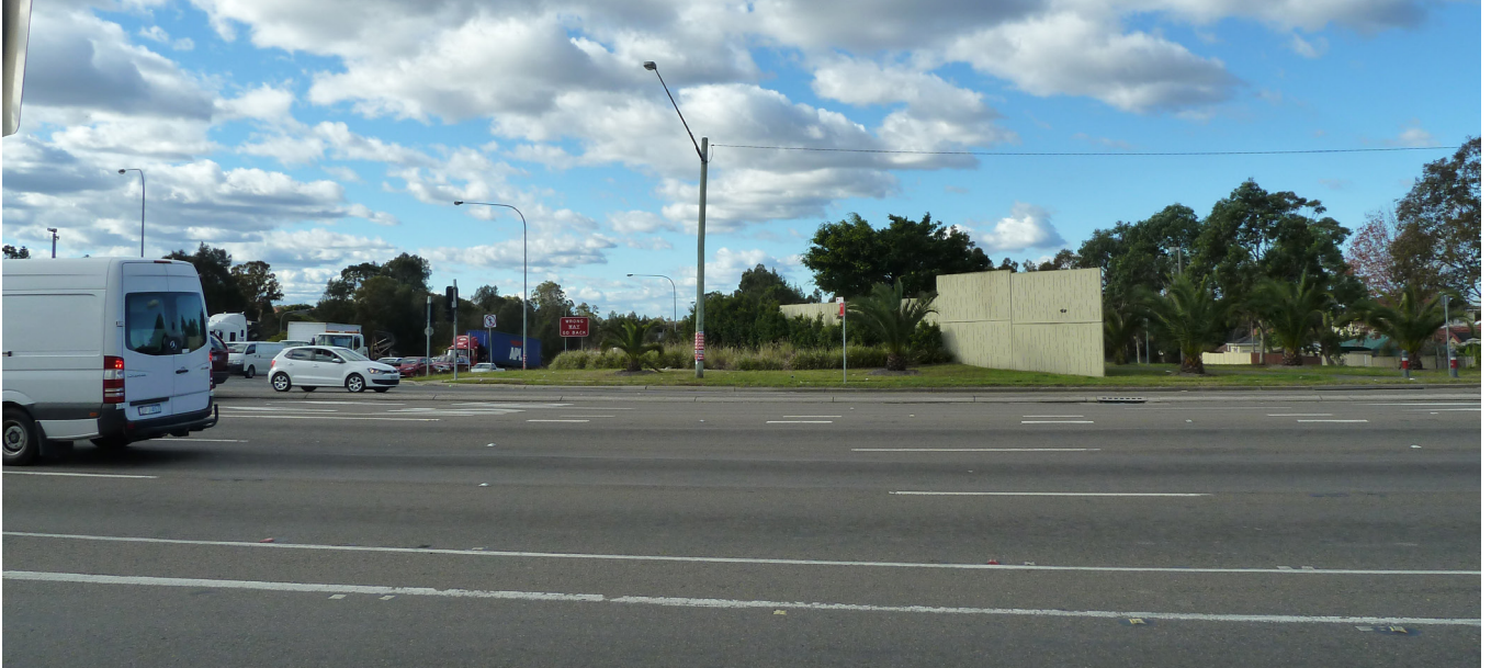
Figure 10 The existing King Georges Road Interchange.
