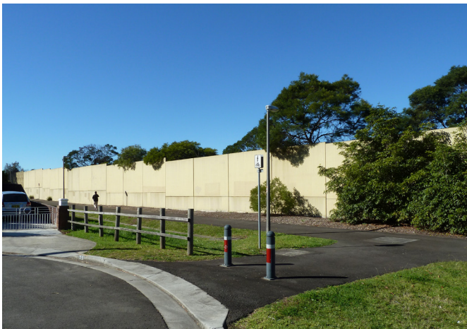
Figure 15 There are 5 different types of existing noise wall within this relatively small project area. These plain panels are adjacent to Kिरrang Street north of the Motorway.
