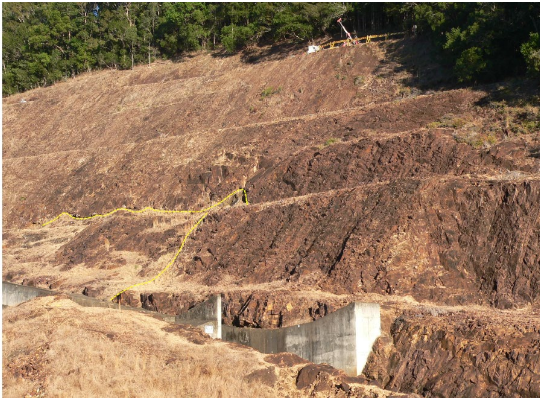
Figure 7.4 Existing benched batter configuration at existing spillway (after NSW PWA 2018a)
