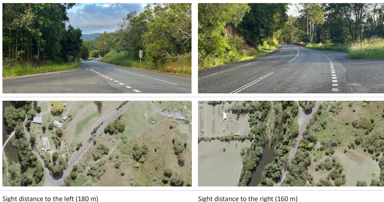
Figure 5.12 Sight distance from Tarcoola Lane to Kyogle Road
