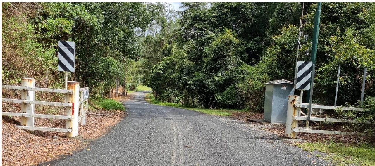
Plate 3.4 Clarrie Hall Dam Road, looking south towards Clarrie Hall Dam
