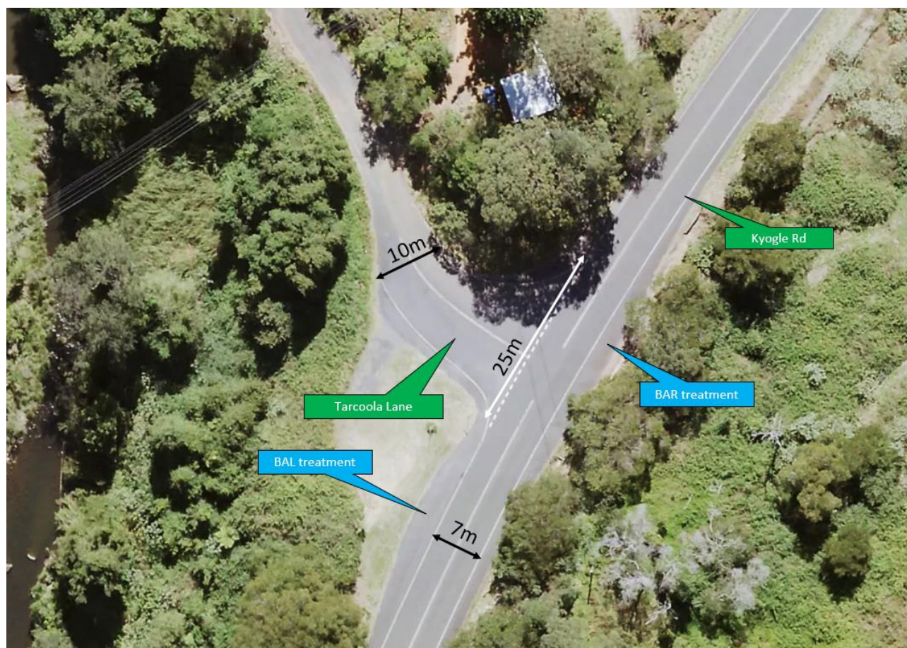
Plate 3.6 Aerial view of Kyogle Road/Tarcoola Lane intersection
