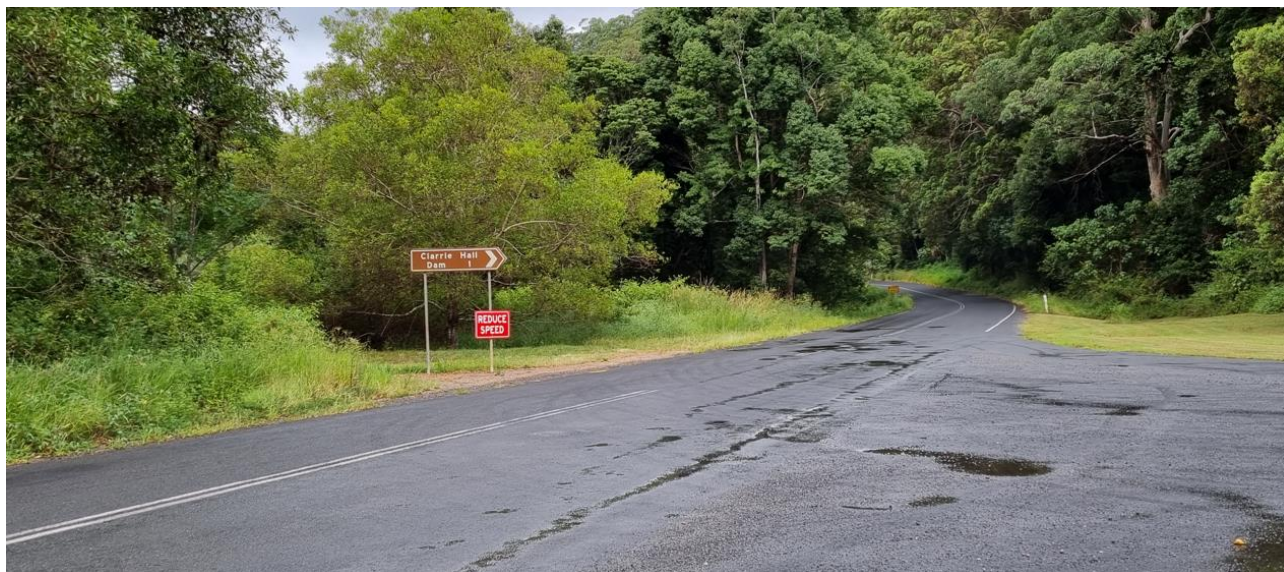
Plate 5.2 Kyogle Road at Clarrie Hall Dam Road (looking east)
