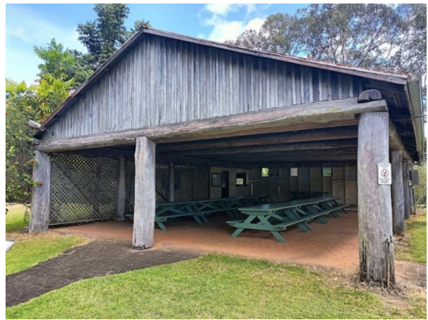
Plate 4.10 Dairy yard from the east showing square notched joinery and refitted interior (Source: EMM 2023).
