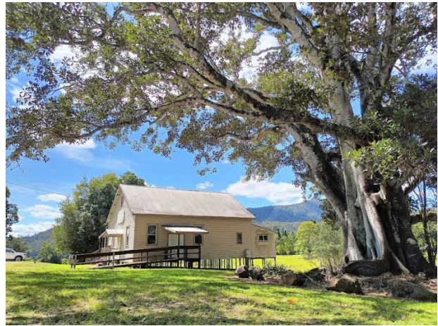
Plate 4.6 View north-east toward Doon Doon Hall showing side ramp and rear additions (Source: EMM 2023)
