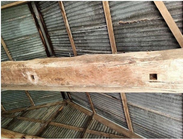
Plate 4.13 Mortise recesses for previous bail yard divisions. (Source: EMM 2023)
