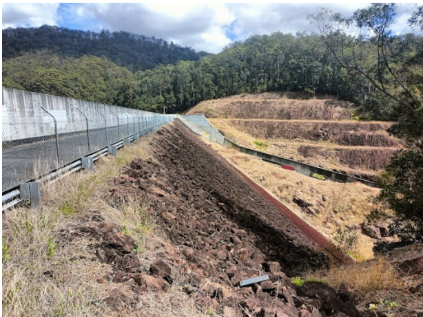
Plate 4.1 View west across the rockfill embankment of the dam toward the distant concrete spillway (Source: EMM 2023)
