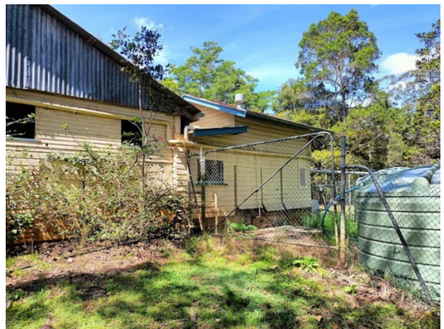
Plate 4.16 View south-east toward dairy/kitchenette addition (Source: EMM 2023).
