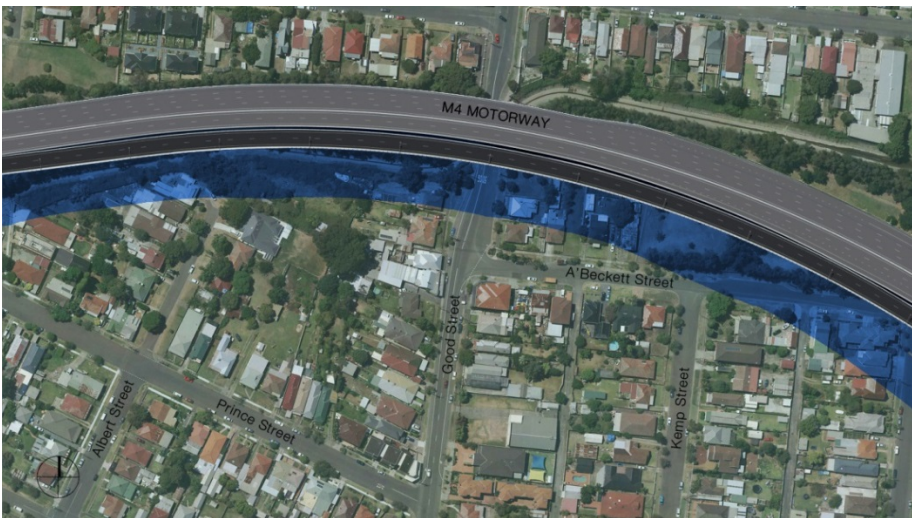
21 June 09:00 – new viaduct
