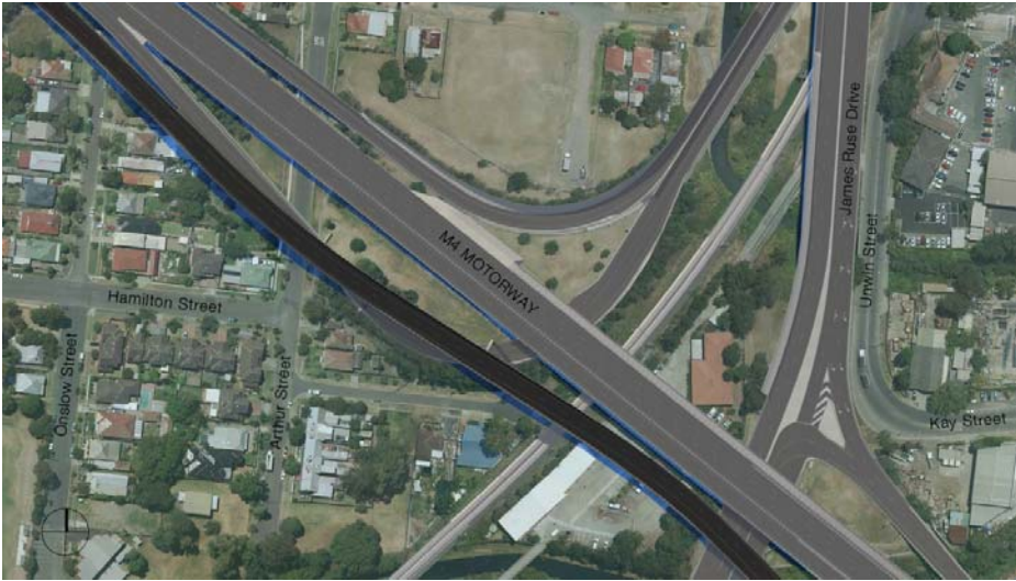
21 December 12:00 – new viaduct
