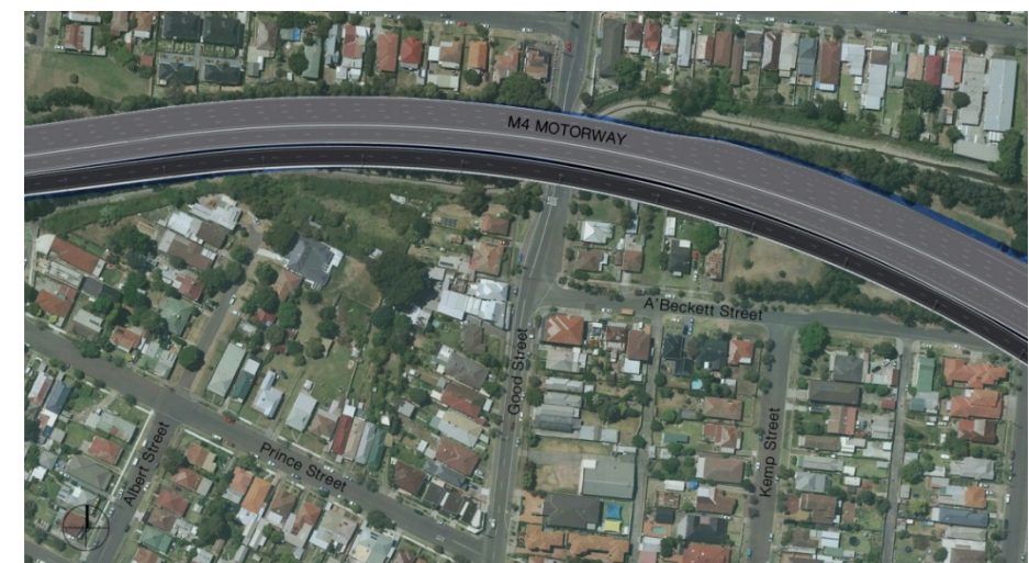
21 December 15:00 – new viaduct
