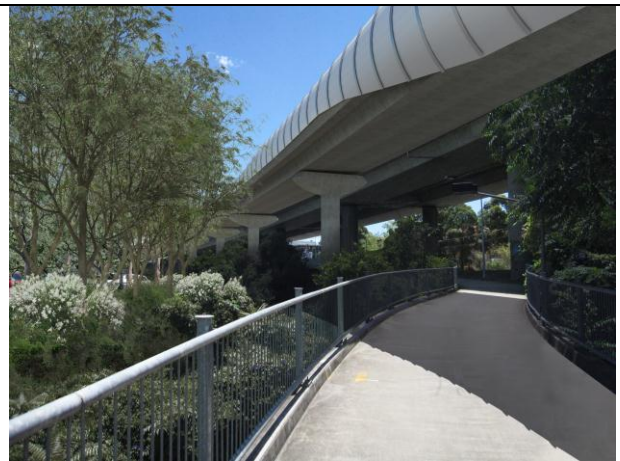
Site photo with viaduct shown indicatively.
