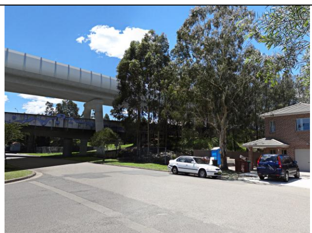
Site photo with viaduct shown indicatively.
