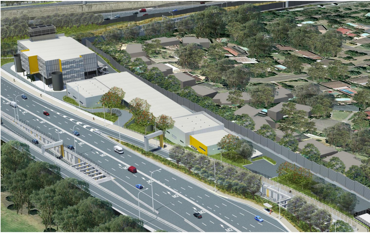
Figure 6-14 View of motorway operations complex - maintenance centre - Pennant Hills Road looking west
