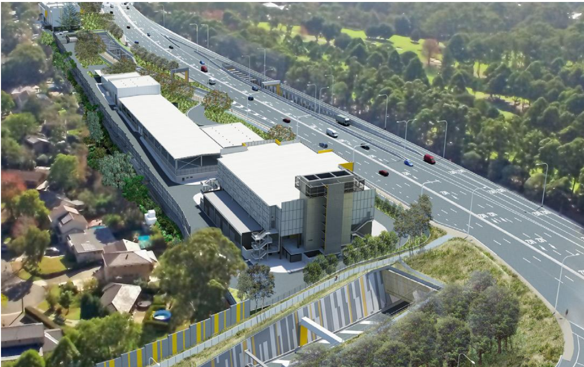
Figure 6-12: View of motorway operations complex - southern ventilation facility
