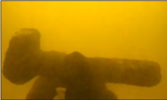
Photograph 30: Bolt or railway spike
