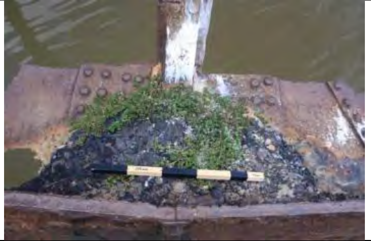
Photograph 26: View of black pitch between stern post and rear bulkhead
