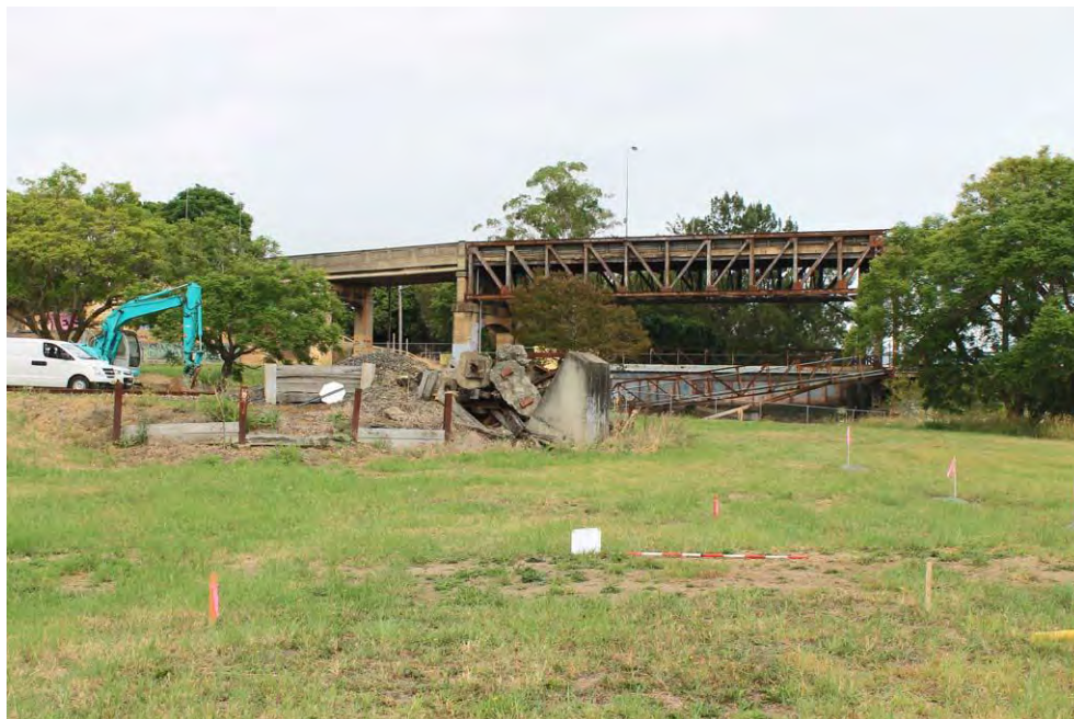
Figure 10: Test Trench 1 looking west prior to excavation.
