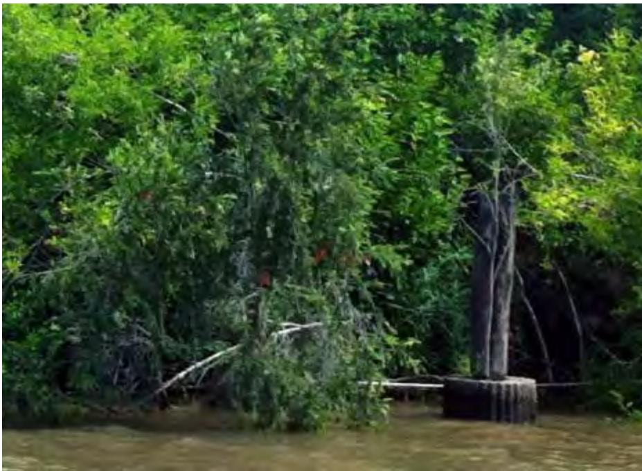
Photograph 15: Exposed remains of timber post with concrete sleeve at base near river bank – showing corrugated outer surface of the sleeve
