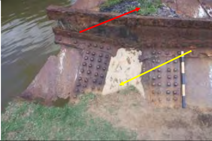
Photograph 25: Detail of stern area showing relationship of concrete (yellow arrow) and pitch (red arrow)
