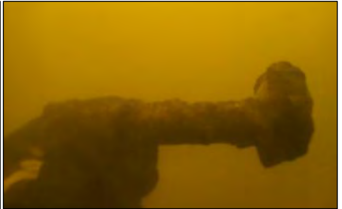
Photograph 31: Bolt or railway spike
