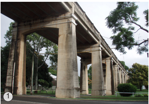
Plate 2.17: Road viaduct, Grafton.
