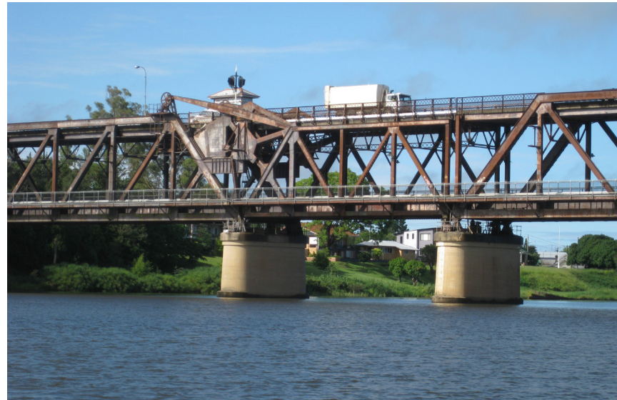
Plate 2.14: Double deck bascule span
