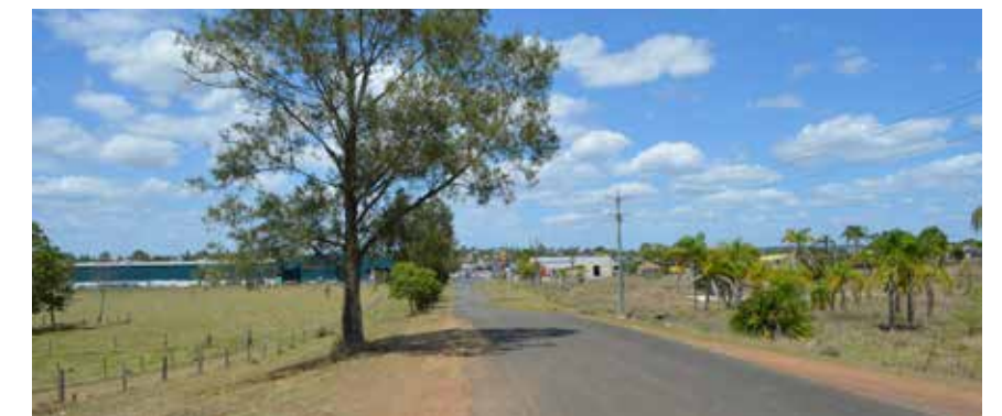
Plate 6.10: View along existing Iolanthe Street, looking south
