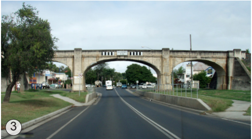
Plate 2.19: Railway bridge over local road, Grafton.
