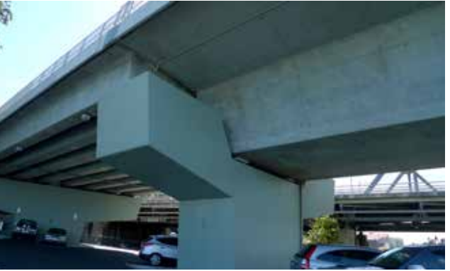
Plate 6.8: Transition pier between box girder and Super T girders at the new Iron Cove Bridge.
