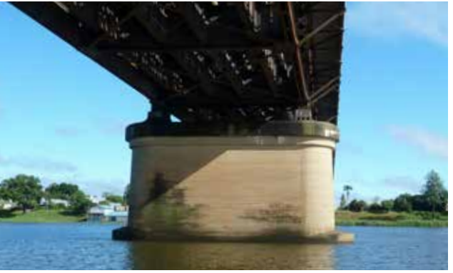
Plate 6.9: Slightly tapering pier shape with rounded pier ends on the existing Grafton Bridge
