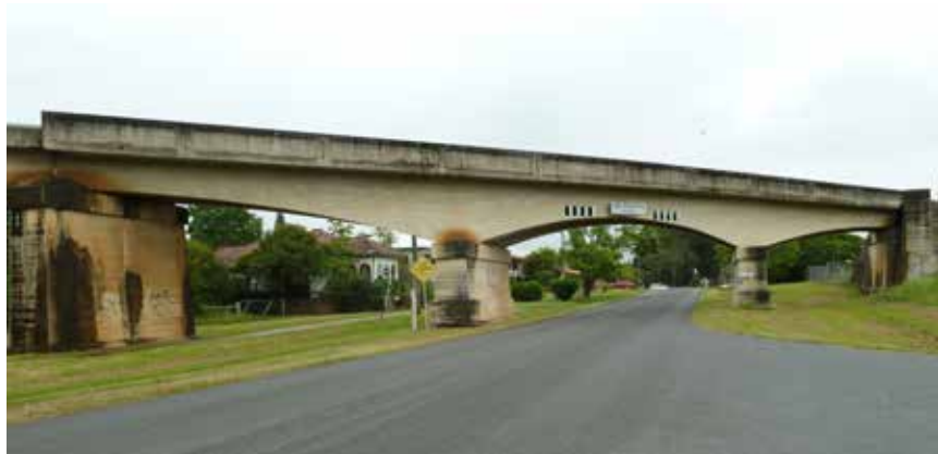
Plate 6.4: Existing railway viaduct over Pound Street, Grafton
