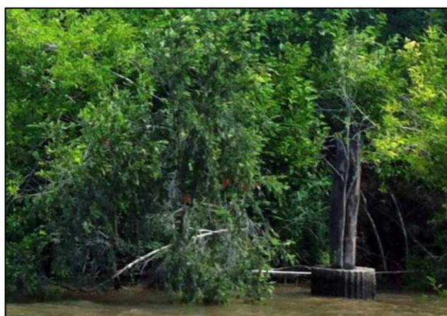
Plate 54: Remains of a timber post (left) and (right) Exposed remains of timber post with concrete sleeve at base near river bank – showing corrugated outer surface of the sleeve (Source: Comber Consultants)
