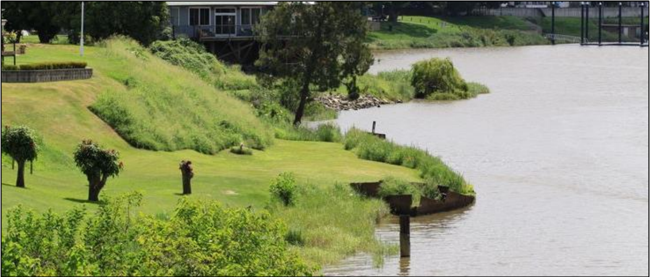
Plate 57: Western facing photograph of the SS Induna (FMW29) which clearly shows the embankment extending over SS Induna hull and the proximity of the existing levee (Source: Comber Consultants).
