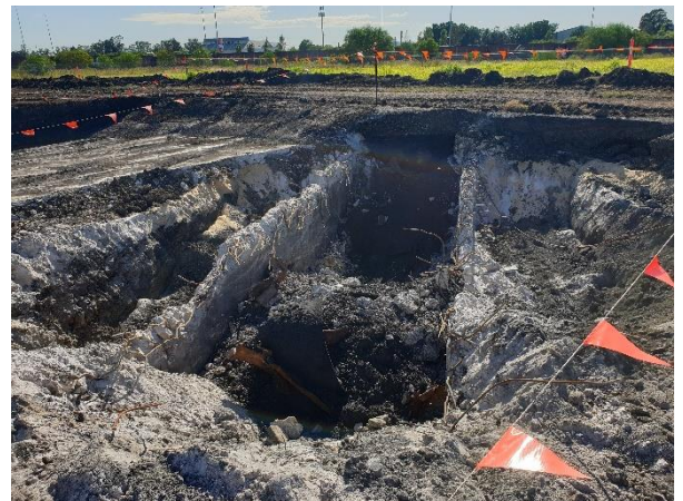
Figure 6: Leg 1 uncovered ROM bin
