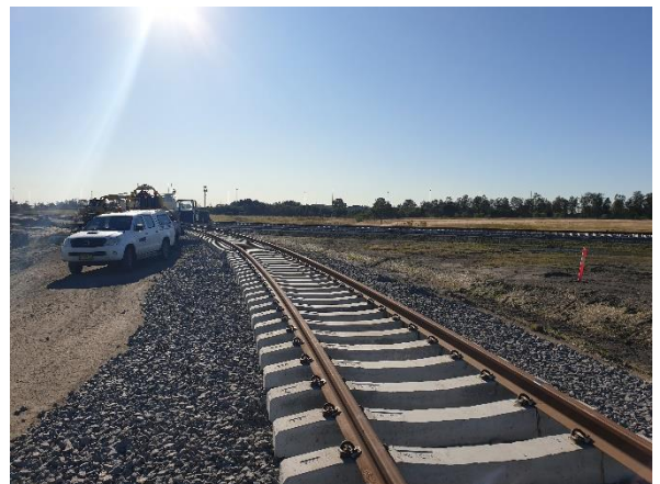
Figure 6: Leg 3 rail and ballast (26/06/20)
