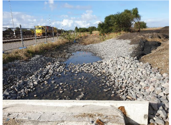
Figure 2: Leg 1 western drainage line culvert (12/06/20)
